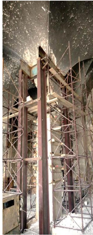
Execute the necessary temporary reinforcement
