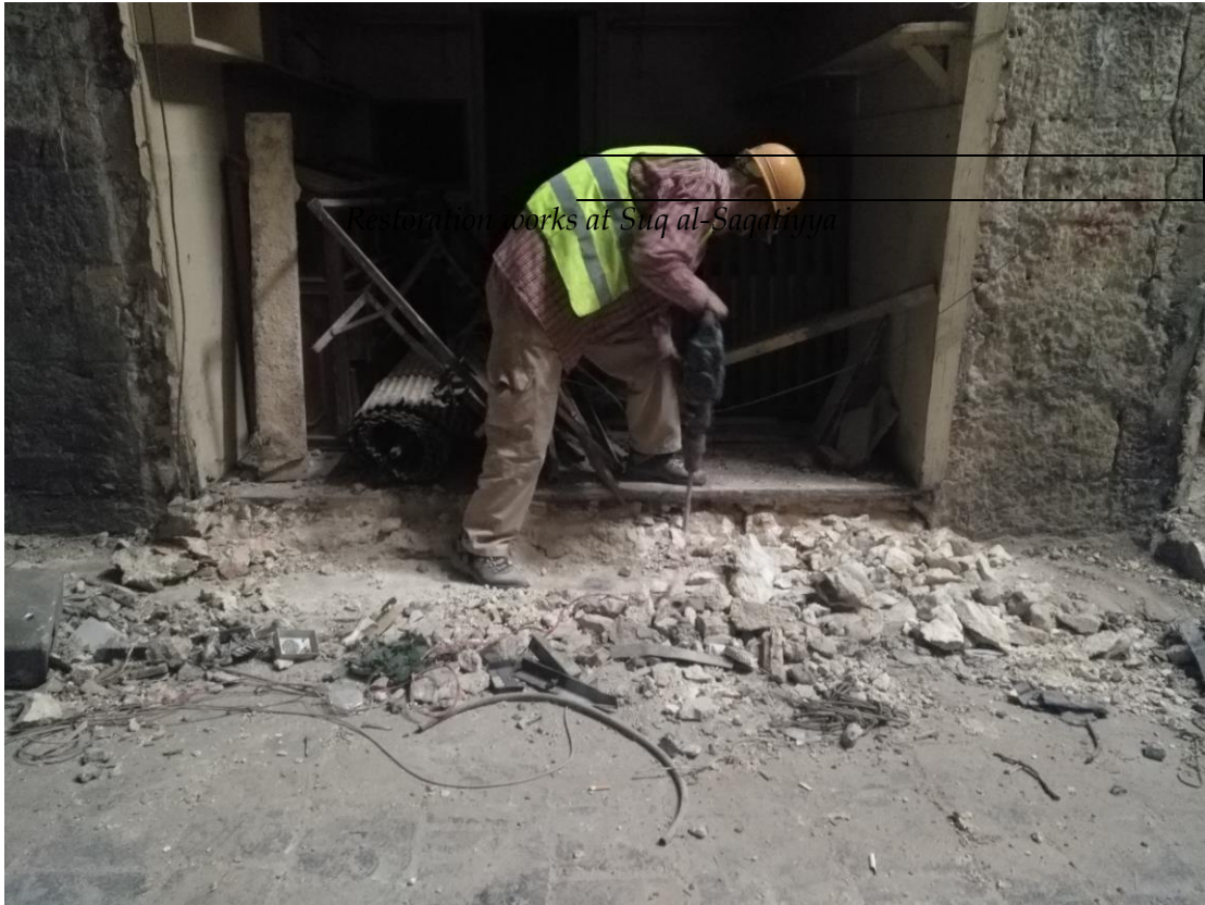
Remove shops entrance threshold at Suq al-Saqatiyya
