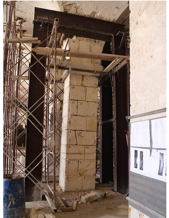
Dismantling the stones and determine the reusable ones for reuse by using the original stones, 95% of the original stones were used, and replacing the remaining quantity with similar modern stones.
