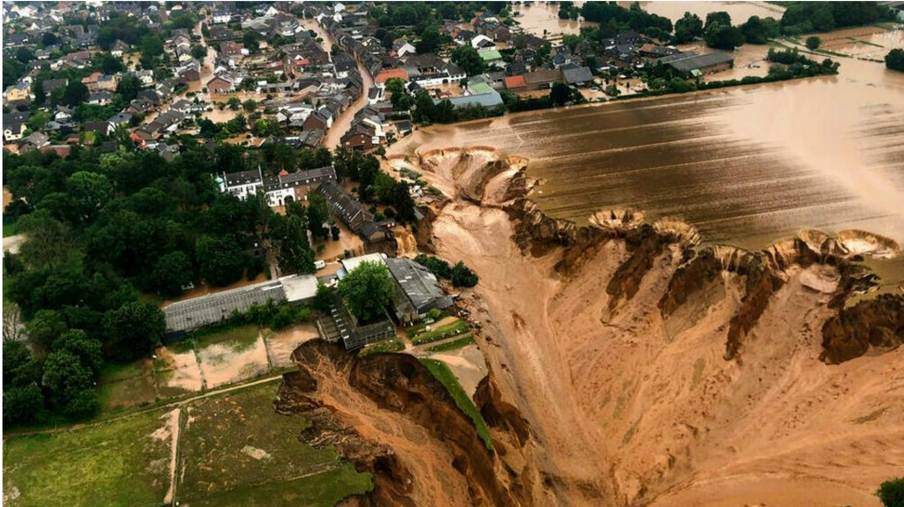
Sinkhole caused by floods in the Blessem district of Erfstadt, Germany. © AP - Rhein-Erft-Kreis
