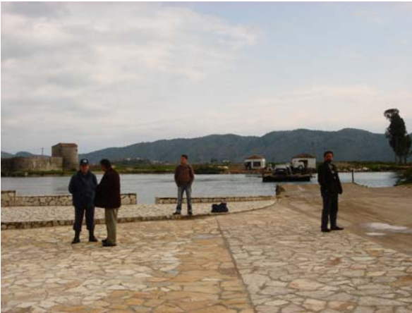
Paving of entry plaza
