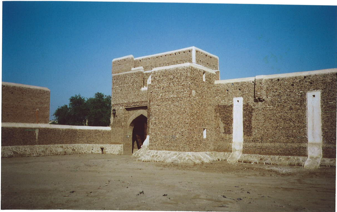
3. Recently Stabilised Minaret and Flanking Wall, and with Adjacent New Building
