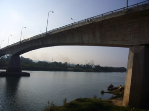
6. The recently built Tuan Bridge, with the by-pass road, has had some negative impact on the nearby Minh Mang and Khai Dinh Tombs
