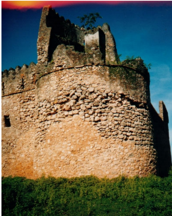
Fig VI d: Gerezza, Damage to wall fabric by weathering
