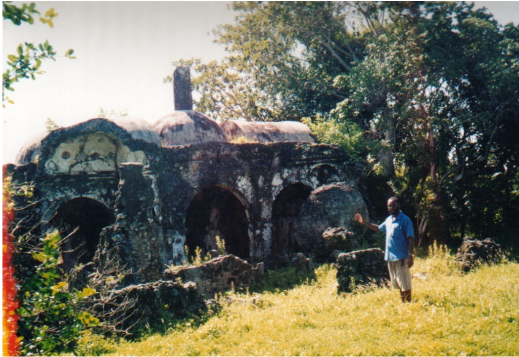
Fig X b: Small domed Mosque with collapsed roof. Outer door pillar collapsing
