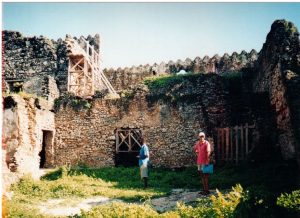
Fig VI f: Gerez, Temporary repairs showing cracks on the left
