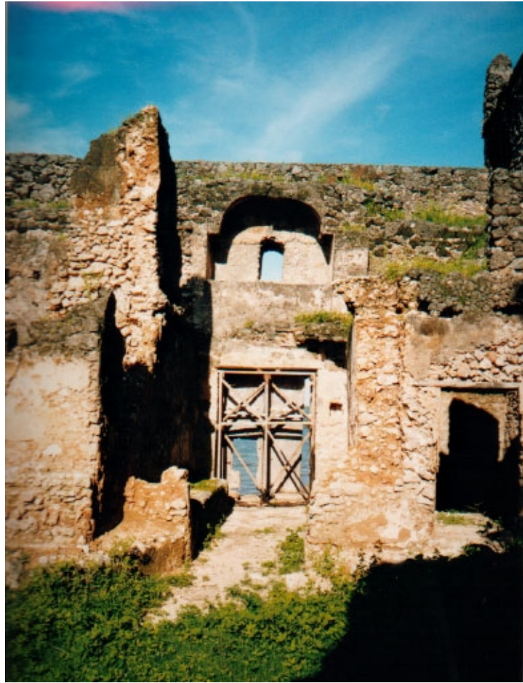
Fig VI e: Gerez, Collapsed arch and flat roof
