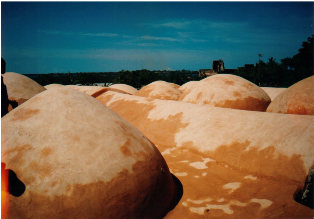
Fig VII d: Great Mosque Roof after renovation combination of barrel vaults and domes
