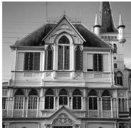
Georgetown's City Hall: an extraordinary example of Gothic architecture in a tropical context, executed in wood with cast-iron elements
