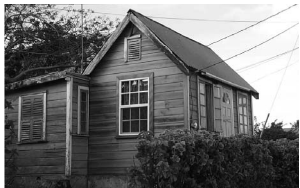
A chattel house in design transition, where there are varying window types: jalousie, sash and double-hung glass. The entrance door is also on the move.
