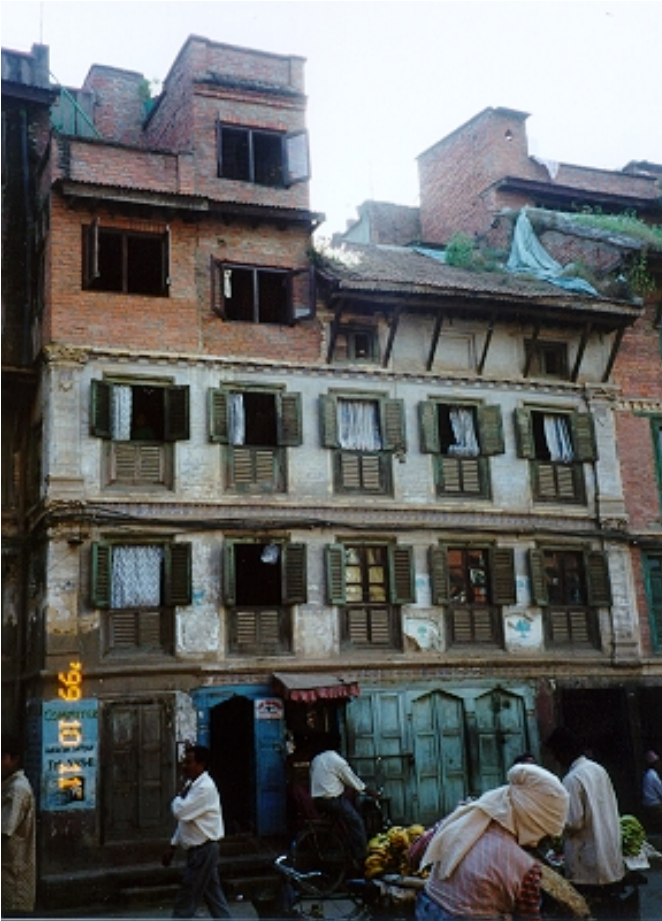
(Above) Two new floors were added in March 1999 after partial demolition of the original sloped roof.
