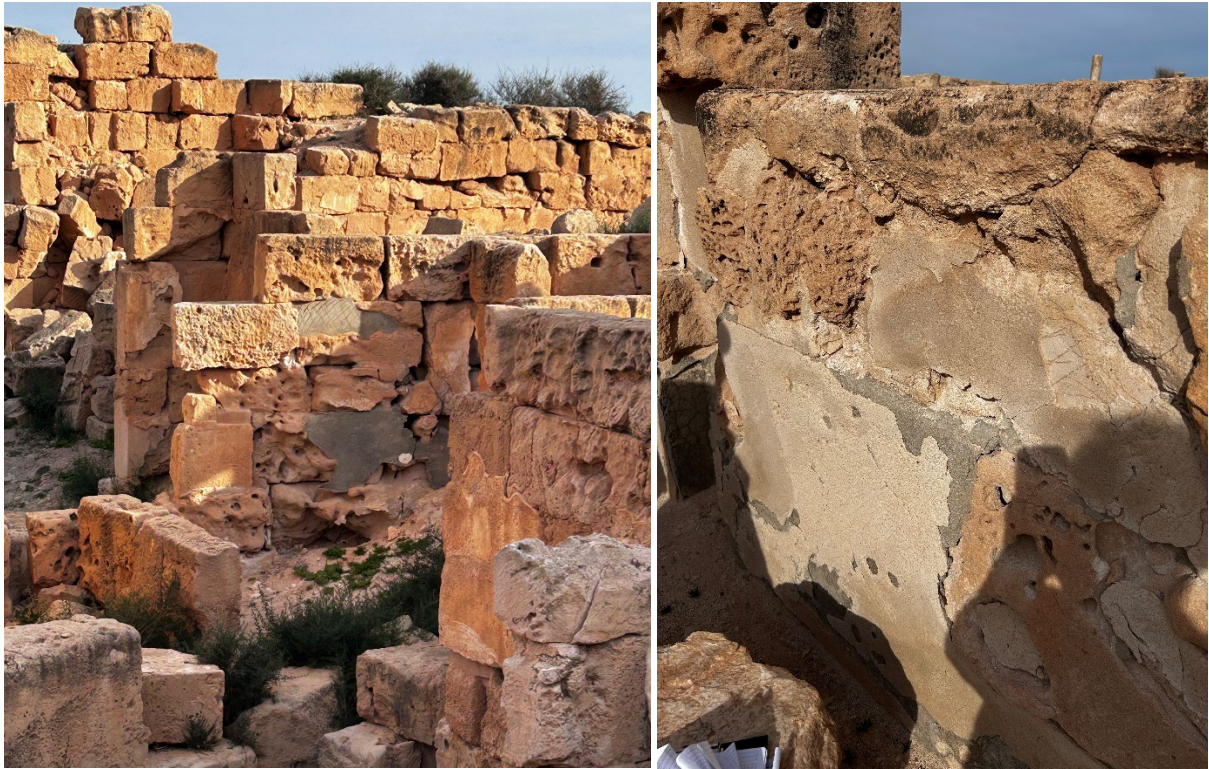
Figures 7 and 8: Previous intervention with the use of cement based mortars© ICOMOS / T. Grandin
