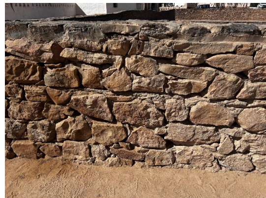
Figures 19-21: Vulnerable structure (left), modern adaptations that could be improved (top right), and example of well-built masonry fence whose coping could have been made with traditional mortar (bottom right) © ICOMOS / T. Grandin
