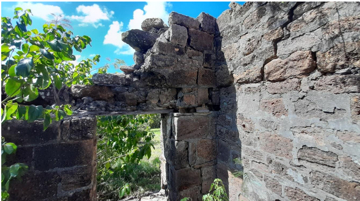
Photo 32: One of the many former military ensembles located within the property. Overall, they show an important deal of decay and deterioration. This particular has severe botanical-related decay and some of its structural components (portion of the wall) are almost about to collapse.
