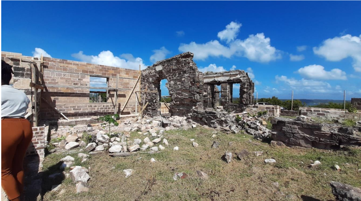
Photo 31: One of the many former military ensembles located within the property. Overall, they show an important deal of decay and deterioration. This particular has severe botanical-related decay and some of its structural components (lintel) are almost about to collapse.
