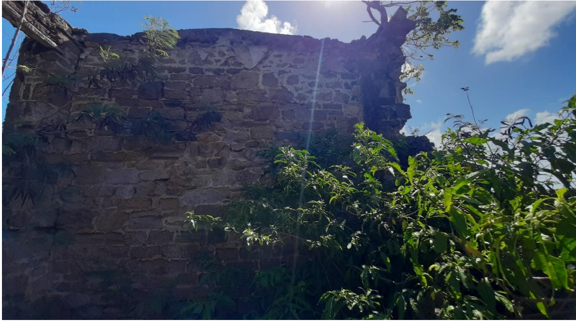
Photo 33: One of the many former military ensembles located within the property. Overall, they show an important deal of decay and deterioration. This particular has severe botanical-related decay and some of its structural components (lintels) are almost about to collapse.
