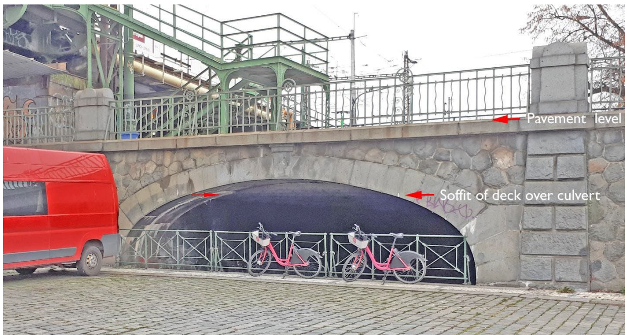
Fig. 16 Mouth of the culvert allowing the Botič Stream to flow into the Vltava (P Drury, 11 December 2024, annotated).
