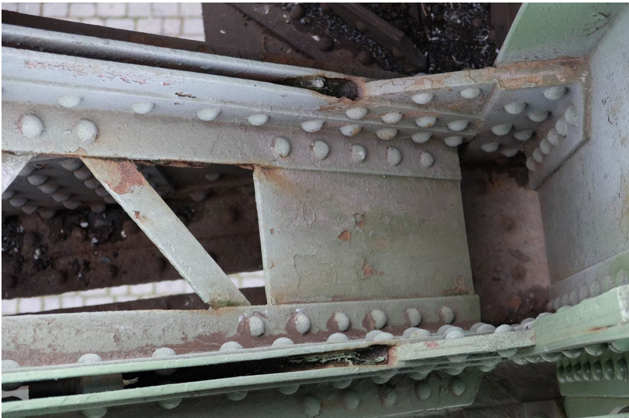
Fig. 9 Typical connection between diagonal, bottom chord and vertical, with angles and gusset plates connected with rivets. (B. Espion, 11 December 2024).
