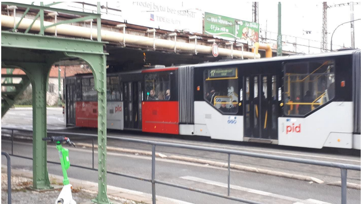
Fig. 15 Limited clearance (presently 3.1 m) under the last span of the viaduct Fig. 1, 2 before the trussed bridge 1 (P Drury, 11 December 2024).
