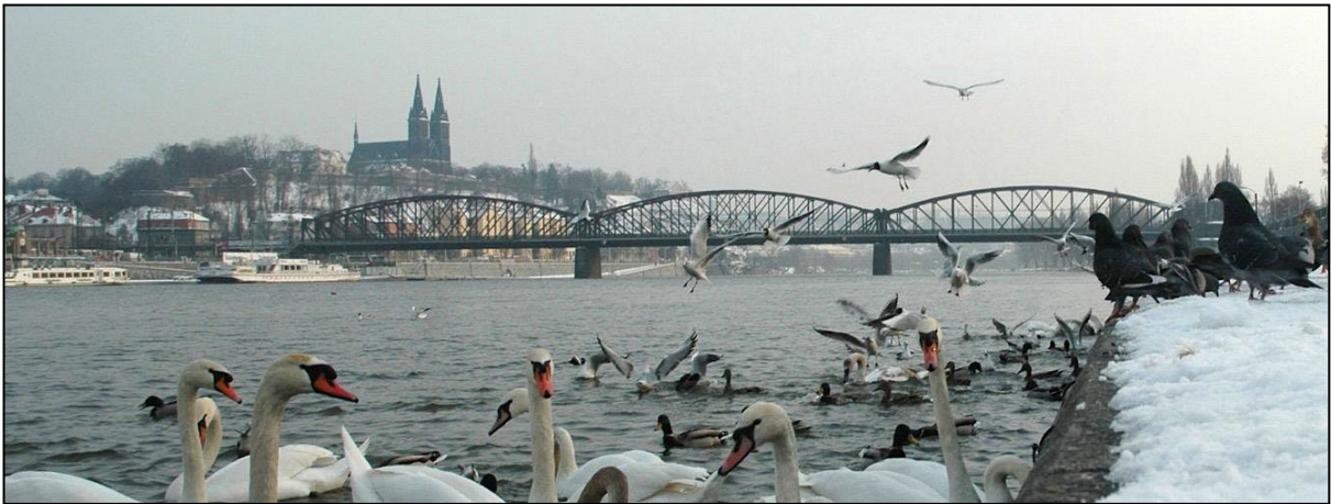
Fig. 5 The bridge, with Vyšehrad fortress and basilica in the background. Note how the appearance of the trusses varies according to the angle of view (NHI, slide 20).
