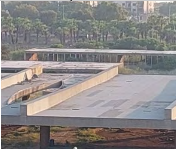
7. Distortions and deflections at the Grand Cover © ICOMOS / G. Stegen
