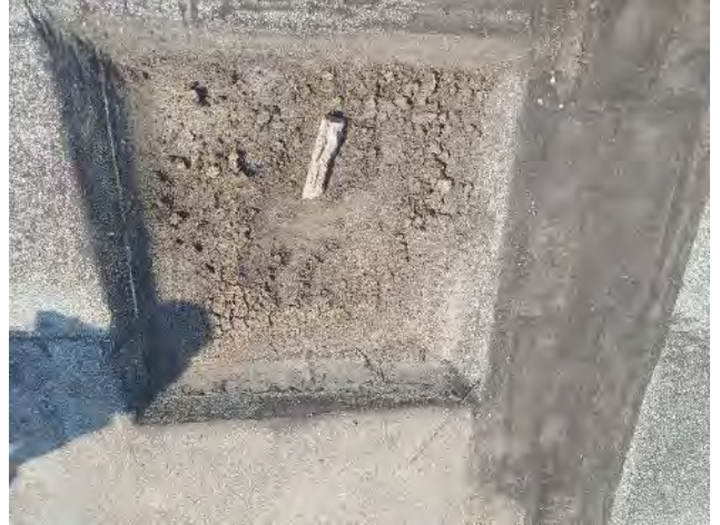
34. Closed roof drains at the Grand Cover © ICOMOS / G. Stegen
