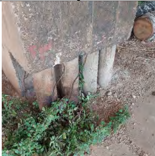
26. Iron rain piping enclosed in the concrete columns- Grand Cover © ICOMOS / G. Stegen
