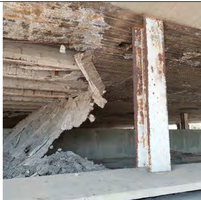
13. Collapse of the soffit at the Open Air Theatre © ICOMOS / G. Stegen
