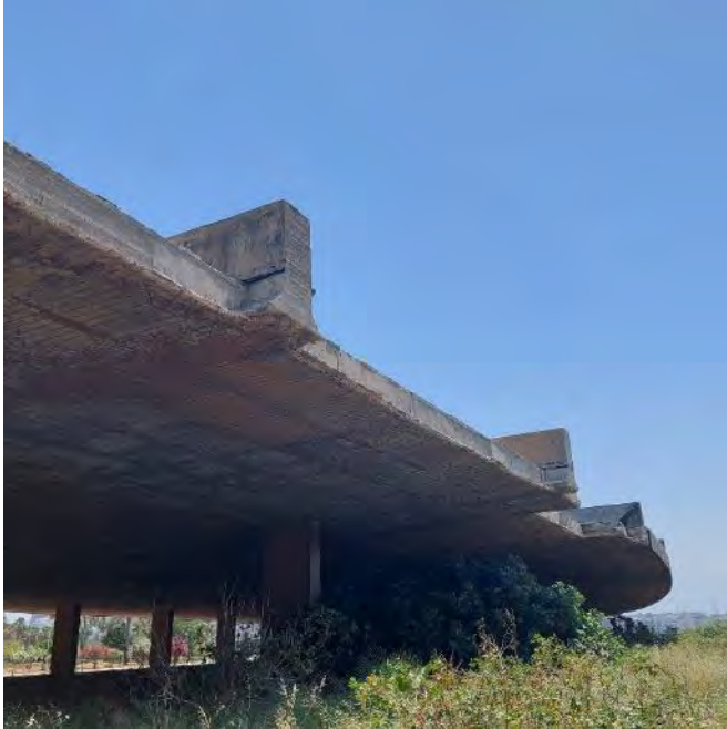
33. Grand Cover- collapse of secondary beams © ICOMOS / G. Stegen
