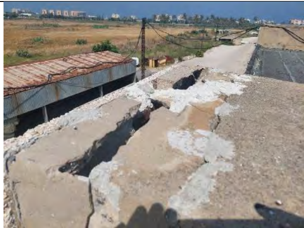
32. Precast concrete facia at the Grand Cover- thickening the edge and moving away © ICOMOS / G. Stegen
