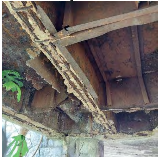
12. Metal lost formwork at a model residence © ICOMOS / G. Stegen
