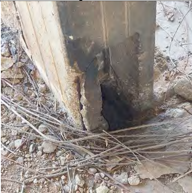
27. Dedicated voids in the formwork- Administration building © ICOMOS / G. Stegen
