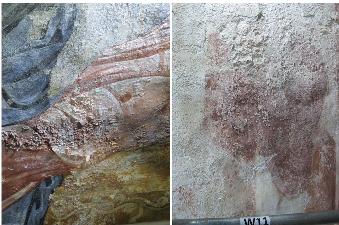
Fig. 3, 4. Flaking, scaling and powdering of paint layer
