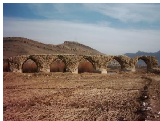
restoration of bridge arches – before
