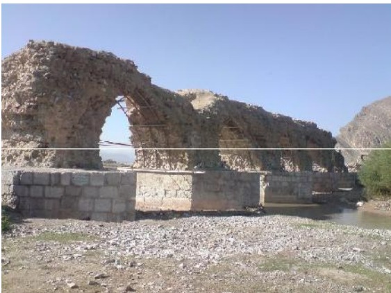
Restoration of the bridge's splashguards(cutwater) - after restoration
