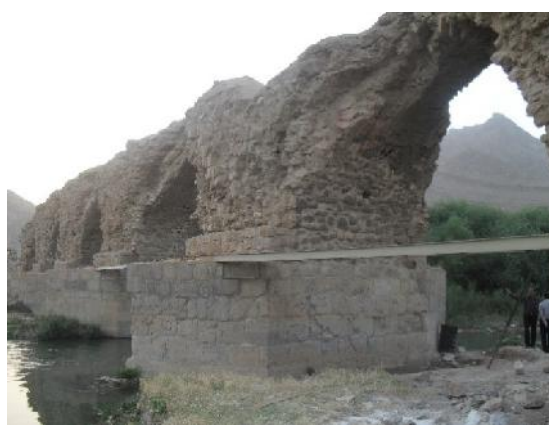
Implementation of the protective structure of arches – before
