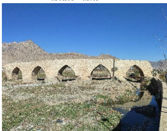
restoration of bridge arches -after
