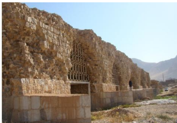
Implementation of the protective structure of arches - after
