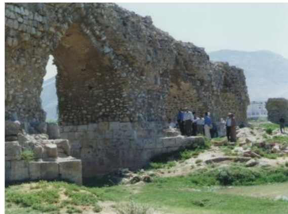
Restoration of the bridge's splashguards - before restoration
