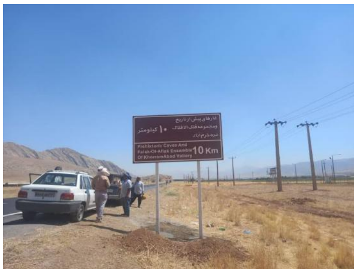
Installation and completion of in-city directional signage
