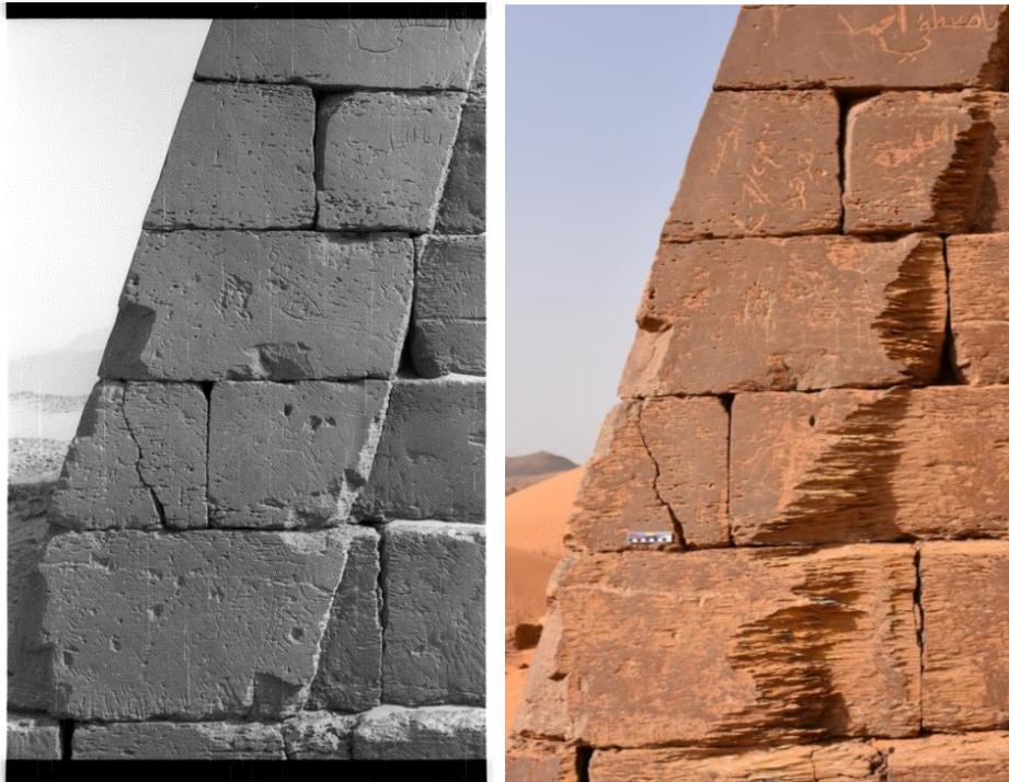
**Sand erosion 1985 left and 2015 right**
