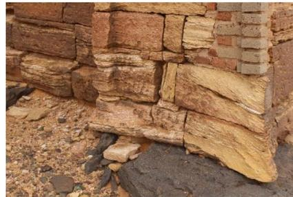
**Sand accumulation and the erosion of corners**
