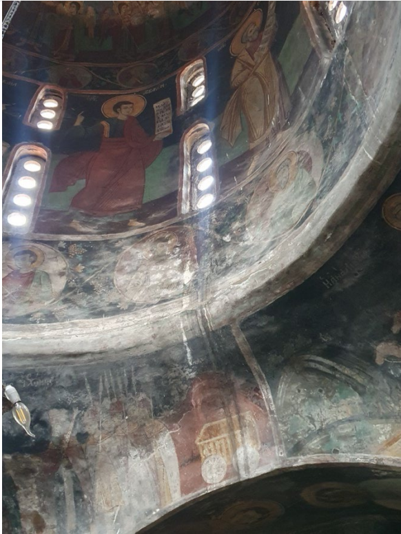
Photo 24 Effects of humidity and water infiltration, soiling
