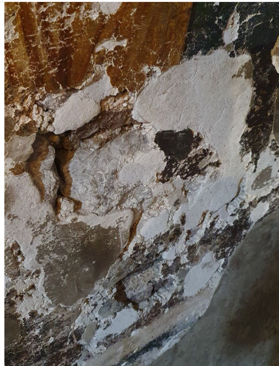
Photo 27 Loss of painted layers and of plaster
