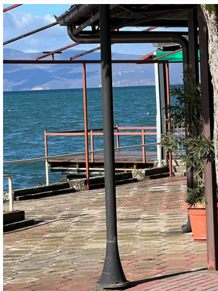
Photo 9 Platform in concrete (fore front), with extension in metal and timber (Ohrid)
