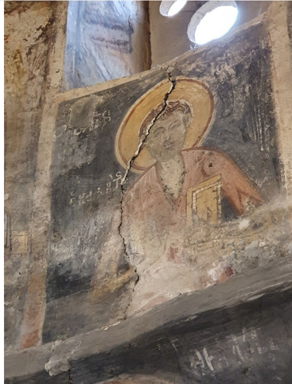
Photo 25 Large crack in the plaster, effects of salt crystallisation
