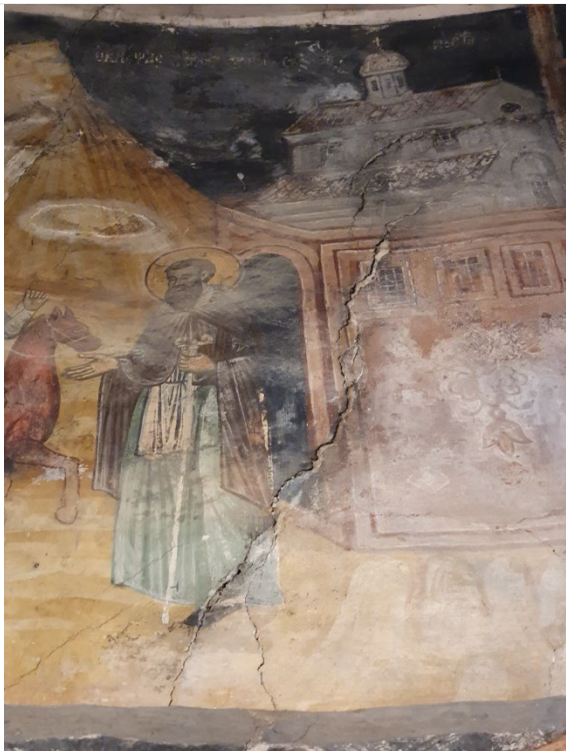
Photo 26 Crack in the painted plaster, effects of salt crystallization on the surface of the paintings
