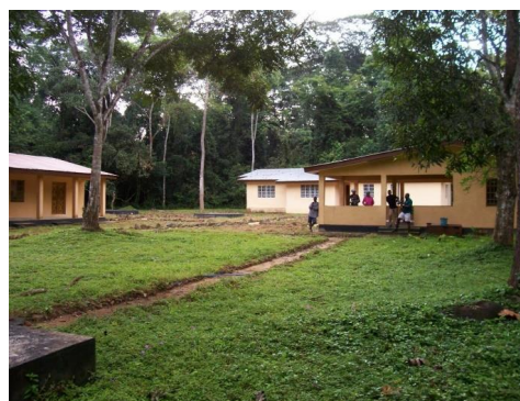
Plate D.4.1 Research Centre Facility at TIWS
