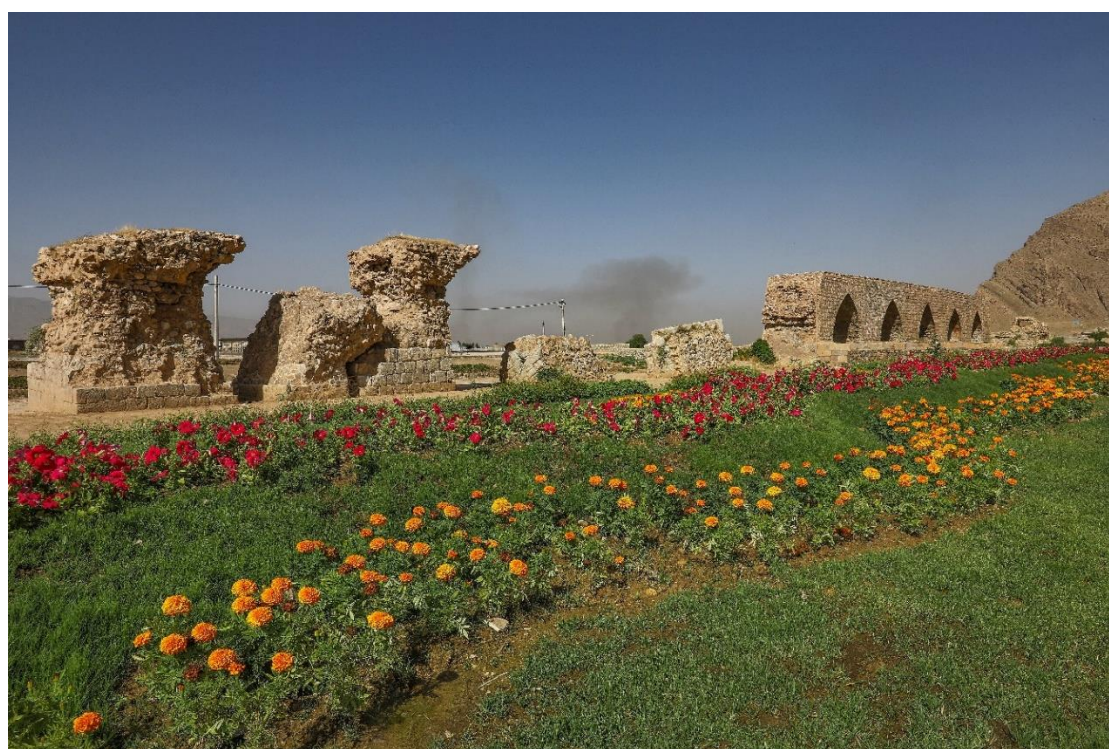
Figure 58: (source: Ali Seifolah Zadeh) Shekaste Bridge
