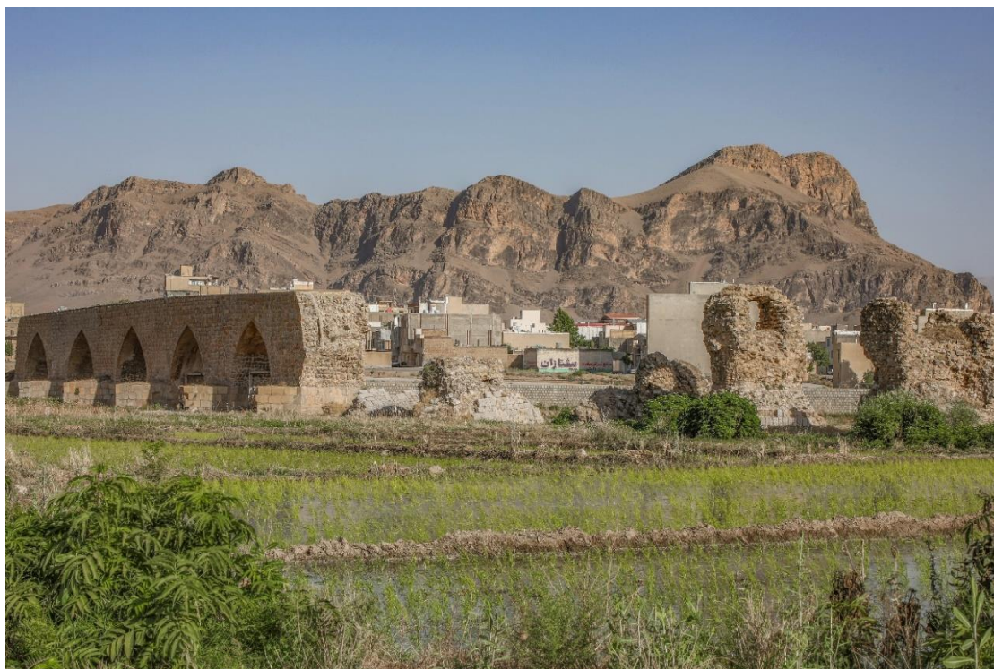
Figure 57: (source: Ali Seifolah Zadeh) Shekaste Bridge
