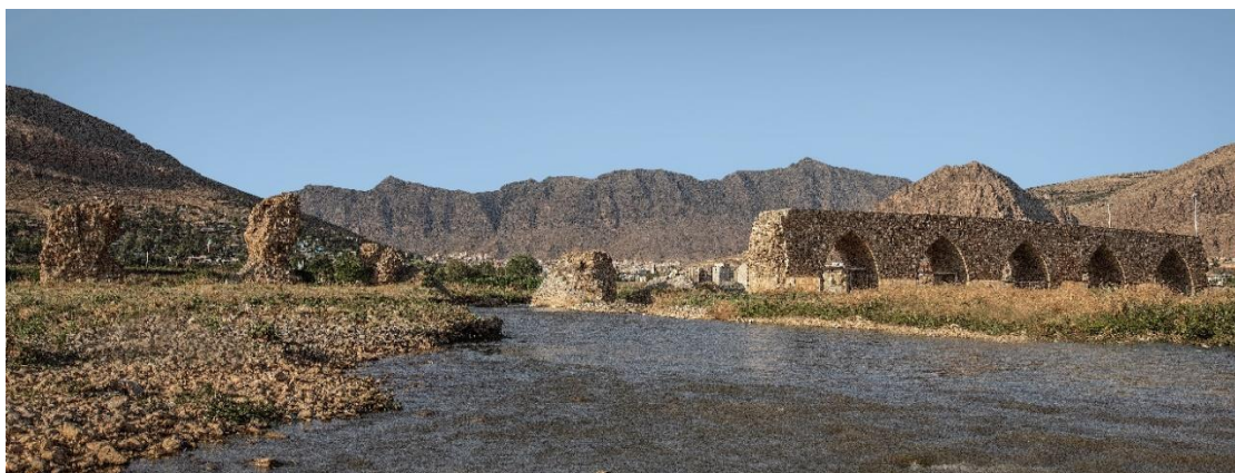
Figure 59: (source: Ali Seifolah Zadeh) Shekaste Bridge
