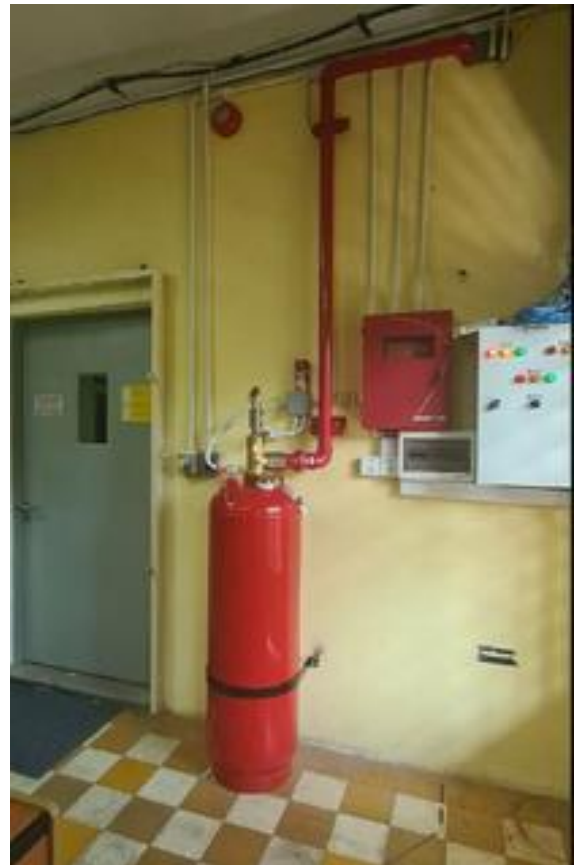
Fire detectors and gas extinguisher system
