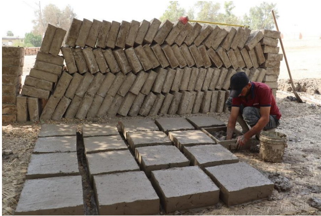
Manufacture the adobe according to the specifications of the original adobe used in the temple
