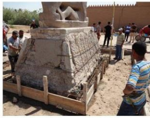
Preparation of the reinforcement of the foundations
