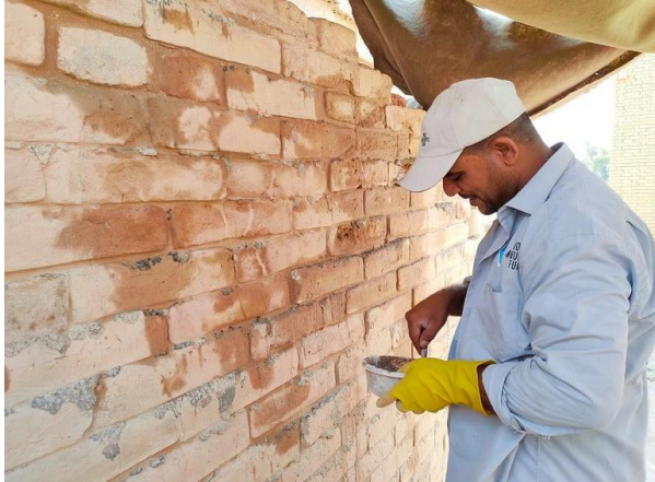
Cleaning and stitching the joints between bricks
