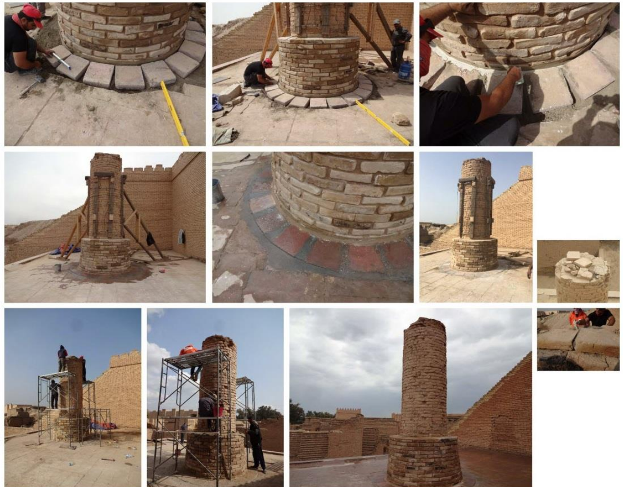
Completion of the pavement, cleaning and repointing of the cylinder, as well as treatment of the top of the cylinder to avoid rain water penetration Cylinder of Al-Madura - Ishtar Gate
