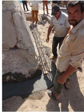
Preparation of the reinforcement of the foundations
