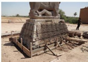
Reinforcement for the new base design as a cage
