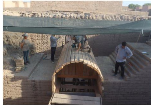
Making a wooden mold for building the arch
