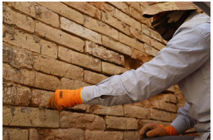
Cleaning and stitching the joints between bricks
