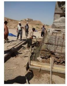
Use of a vibrator for the foundations
