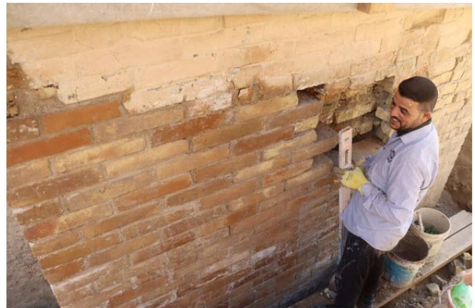
Still damp from installation, a portion of the east flank masonry underpinning was completed before technicians undertake joint pointing. Once dry, the masonry becomes an improved complement to the dimensions, color, and texture of the historic masonry above. September 21, 2023.
