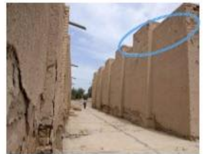
3. Direct weathering on the surface and on the top of walls due to rain and wind
