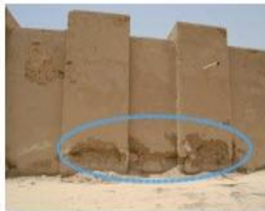
2. Decay of the wall base due to combined action of rising damp and salts (undercut)
