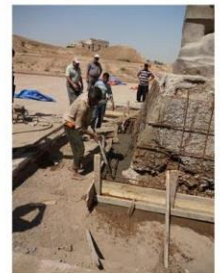
Reinforcement for the new base design as a cage
