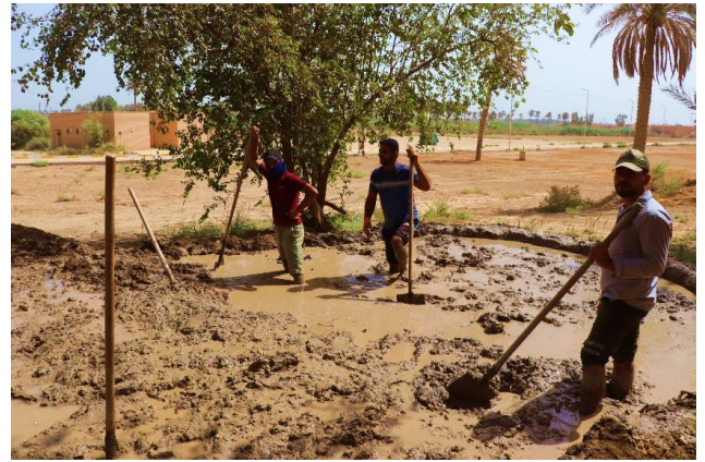
Manufacture the adobe according to the specifications of the original adobe used in the temple
