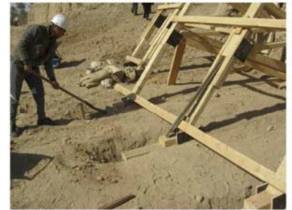
Fixing the base in the ground
