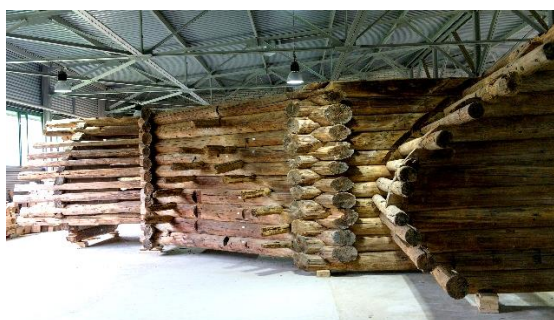
Image 10. 2016. The Church of the Transfiguration during its conservation intervention. Tier 6 has been disassembled from the church, repaired and assembled in the workshop to check for each detail and test loads. Later it was disassembled again, taken to the church and assembled in place.
