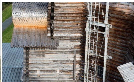
Image 8. 2016. The Church of the Transfiguration, during its conservation intervention. A tier has been disassembled and is being repaired in the workshop. The lower part has already been intervened, with the upper part waiting its turn.
