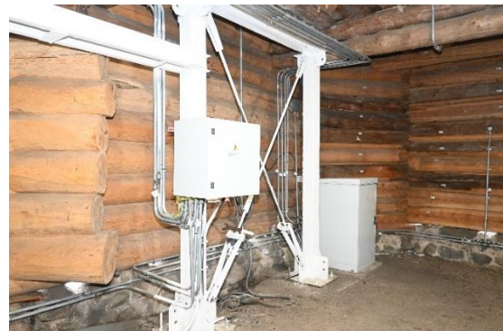
Images 27-28. Fire extinguishing systems at the base of the Church of the Transfiguration - Insulation of the electric power supply system.
