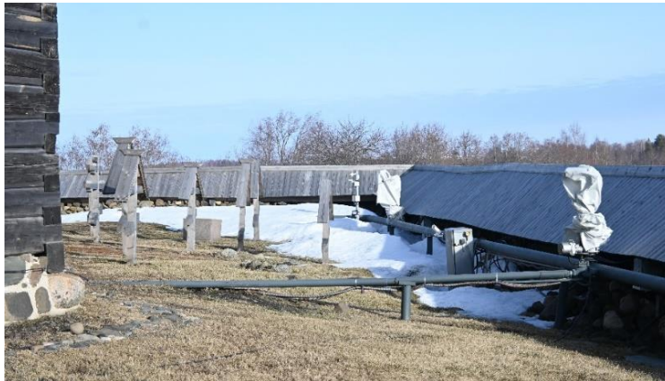
Images 24-25. The existing fire extinguishing and surveillance systems in the yard of the “Kizhi Pogost” World Heritage property.
