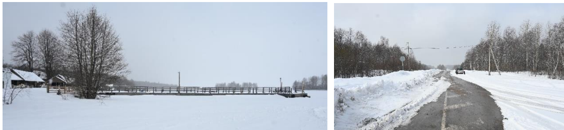
Image 44. The overhauled and put into operation wooden pier.
