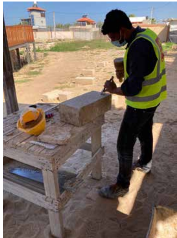
Fig 10: Block cutting and laying (PUI)
