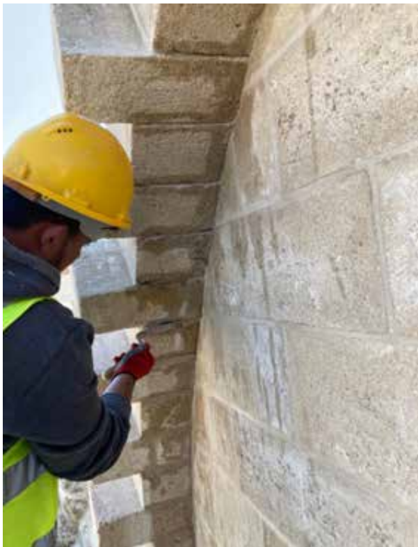
Fig 9: Making mortar joints (PUI)
