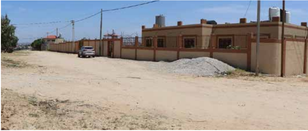
Fig 43. The unpaved street at the main entrance with no spaces designated for parking (PUI)
