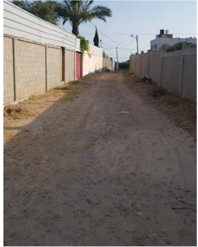
Fig 27. Eastern street 10m on the municipality plan but on the ground is 5m (CCHP 2023)
