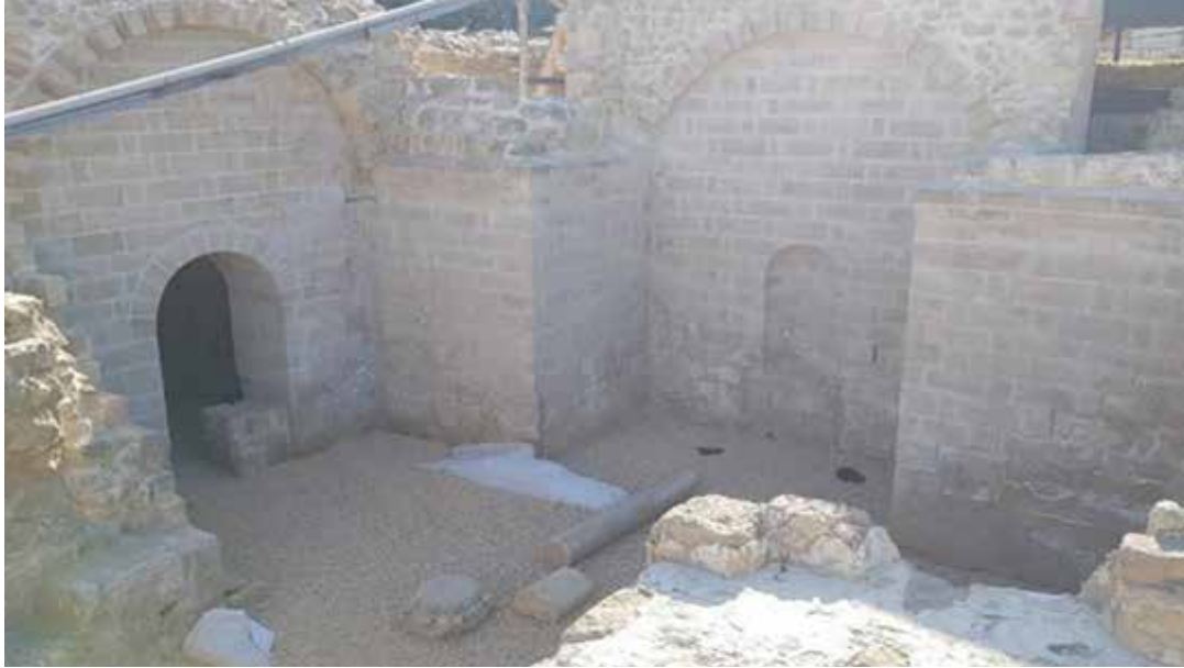
Fig 46. On-site restoration and conservation work (the crypt) (CCHP team 2023)
