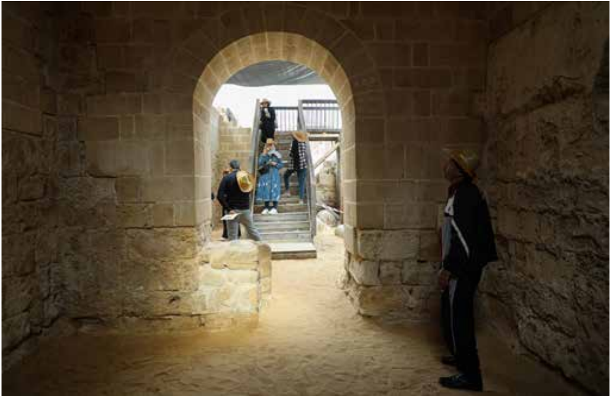
Fig 11: Reconstruction as consolidation work to the main chapel (PUI)
