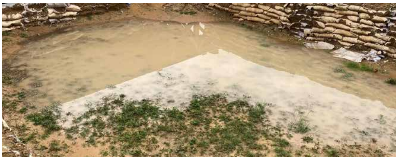
Fig 28. Some aspects of deterioration affecting the Site (R. Elter/PUI)
