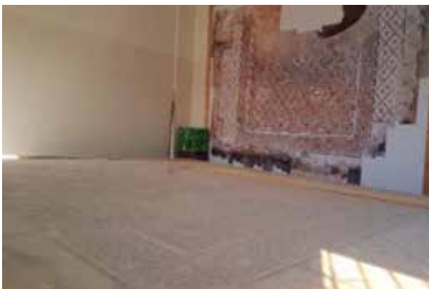
Fig 32. Mosaic restoration works (PUI)
