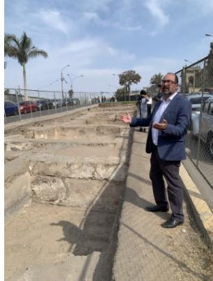
Findings of foundational times: the old Aliaga Mill
