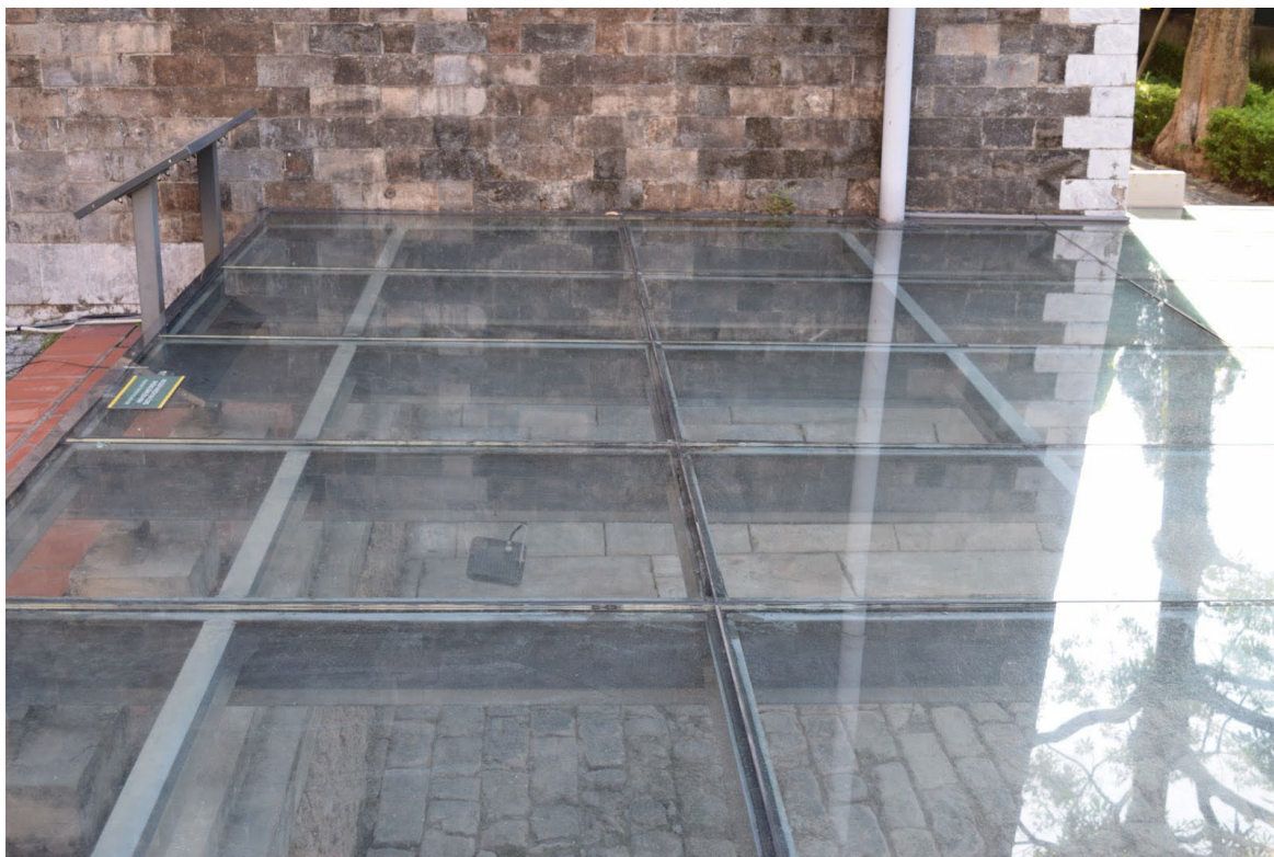
Detail of the steel and glass structure built to protect but leave visible the archaeological findings near Doan Mon Gate. © Luisa De Marco
