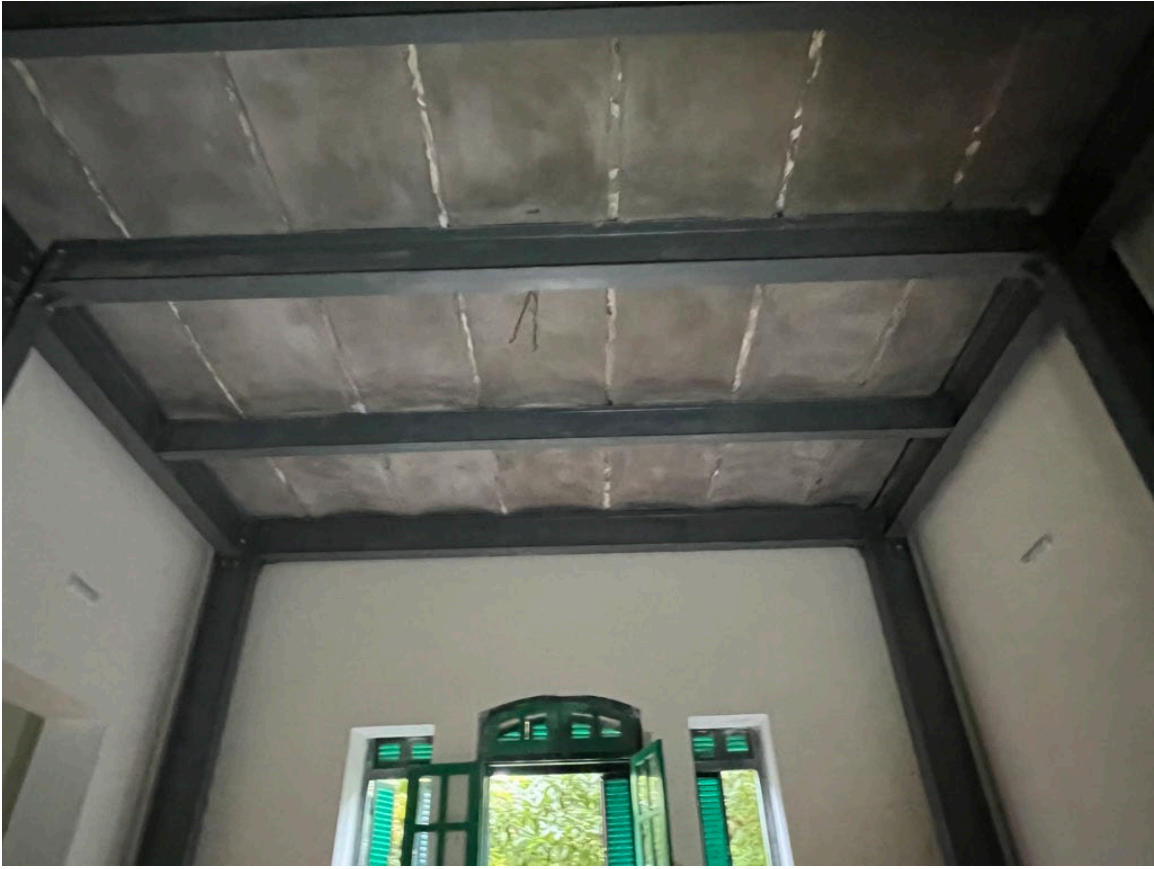
Vaxuco Building. Structural reinforcement with steel beams.
