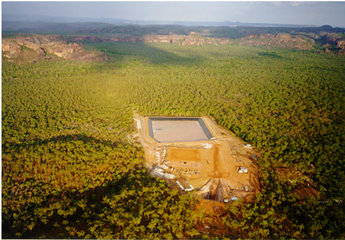
Photograph 1 Aerial view showing the status of the construction of the uranium mine on the Jabiluka Mineral Lease, October 1998.
