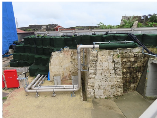
Temporary structures and services have been provided to enable the reconstruction of the replica buildings. These have been designed and installed so as not to impact the significant attributes (archaeology, ramparts) of the site and will be removed on completion of the work. © C.Forbes 2023
