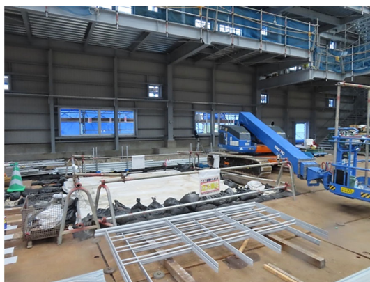
The archaeological remains that were damaged in the fire have been stabilised and covered with temporary protective layers for the reconstruction of the Seiden. The ground surface and archaeology beneath are protected from vehicles and heavy equipment by large steel plates. © C.Forbes 2023
