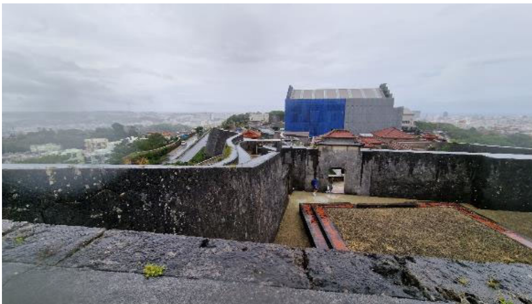
A large shed has been erected over the site of the Seiden to protect it during reconstruction. View from the highest point of the site. © Rohit Jigyasu 2023
