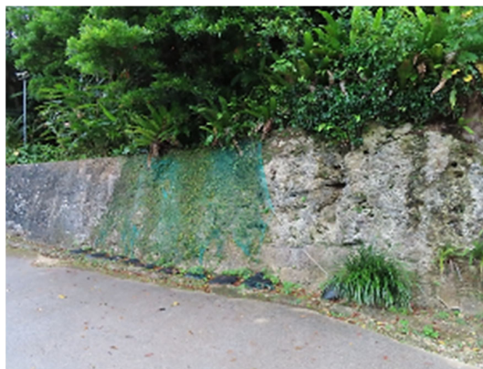
Sections of wall failing due to groundwater pressure have been temporarily stabilised and are to be repaired and site drainage issues resolved. © C.Forbes 2023
