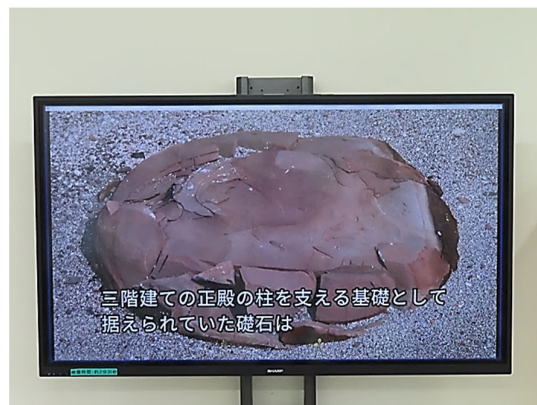
Image from a video display on the site showing the damage to the foundation stones. These have since been ground by community volunteers to enable the material to be used as a base coat for the lacquer to be applied to the reconstructed building. © C.Forbes 2023
