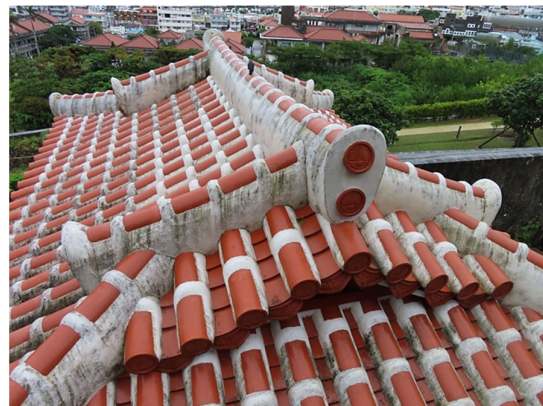
The roof on one of the surviving buildings on the site shows the traditional use of lime mortar to make the tiles weathertight. © C.Forbes 2023
