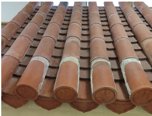
Roof tiles that survived the fire have been salvaged and cleaned for reinstatement on the reconstructed building. © C.Forbes 2023
