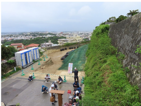
New water tank being excavated adjacent to castle to provide backup supply for future fires. © C.Forbes 2023
