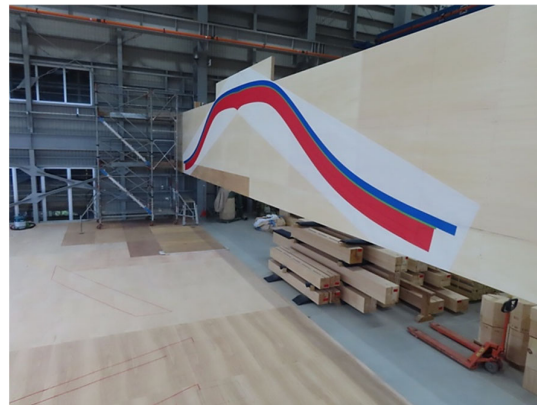
Full scale drawing of curved gable end to be reinstated over the entrance to the Seiden. © C.Forbes 2023
