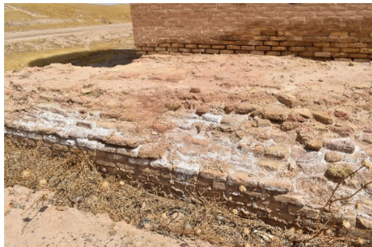
Figures 10 and 11: Al-Ma'shuq Palace, evidence of humidity (left) and slat efflorescence (right) © ICOMOS/Y. Makaroun
