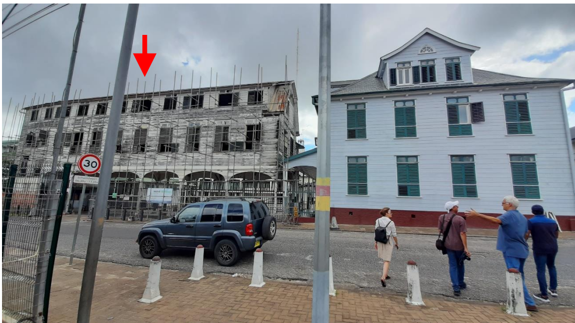
Photo 32: Typical wooden buildings (along Monseigneur Wulfingstraat ) showing advanced state of decay and deterioration (red arrow).
