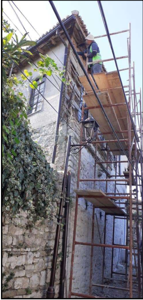
Fig. 9 During the works
