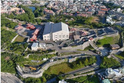
Figure 1 The temporary roof (south side)
