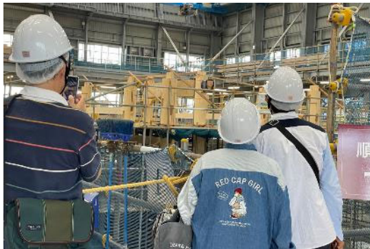
Figure 3 Reconstruction site open to the public
