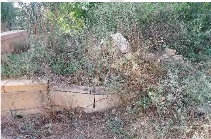
Figure 35 Of particular concern is the subsidence of the surface masonry that makes up the main platform. By all indications, there exists an underground vault that requires structural stabilization. During the monsoon, many other tombs with platforms suffered from near collapse as these vaults were unknown. This situation should be investigated immediately.
