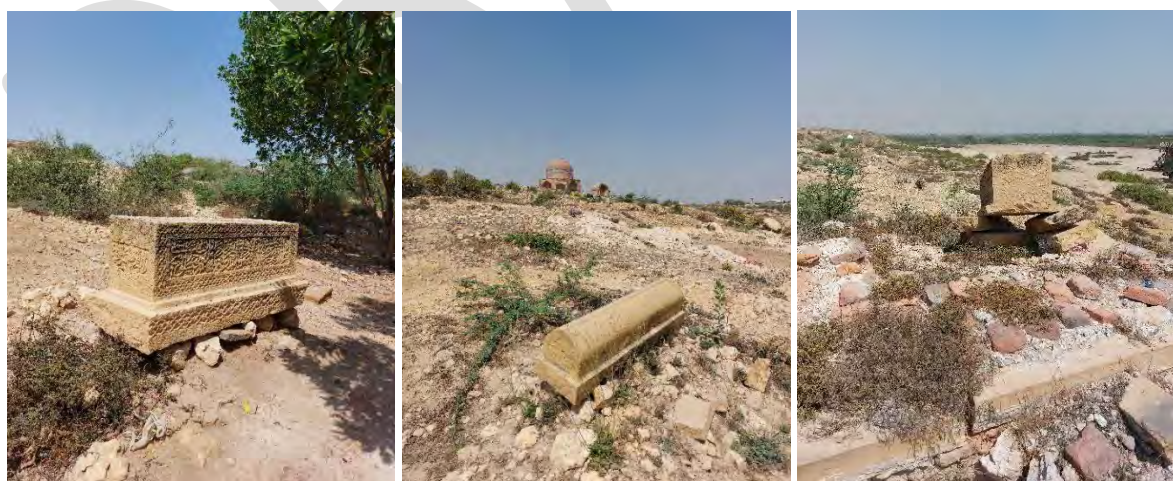
Figure 25 Other small unknown tombs that have been displaced by the monsoon. Most are constructed without mortar on rubble masonry platforms. Fortunately, the masonry platforms can be restored, and the markers reassembled anastylosis. Right, there are other damages, such as the erosion of the platforms that expose the graves below (Eppich).
