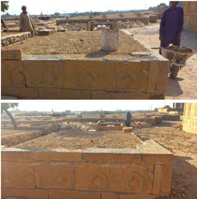
Figure 5 Restoration of a cut stone platform tomb near the monumental tomb of Isa Khan II that was damaged in the monsoon. Above, before, below after (Serfraz Nawaz)
