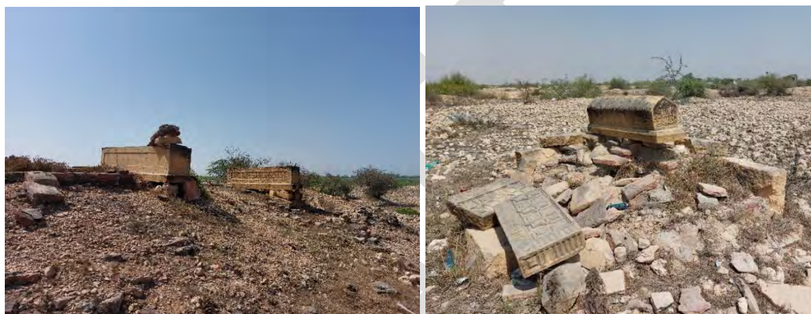
Figure 24 Small unknown grave markers at the eastern edge of the site. Many of these smaller grave markers were displaced during the 2022 monsoon due to unstable geology and heavy rains. These are some of the most vulnerable elements at Makli as they are small, not monumental, and often go unnoticed (Eppich).
