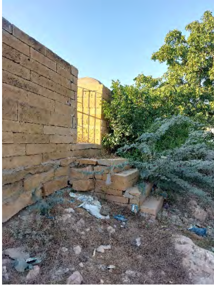
Figure 28 Continued erosion of the access steps and eastern boundary wall of the enclosure tomb of Badi Uz Zamman Tarkhan, left. Right, a 3D model was created of the enclosure tomb of Amir Habshad Bai to document the erosion.
