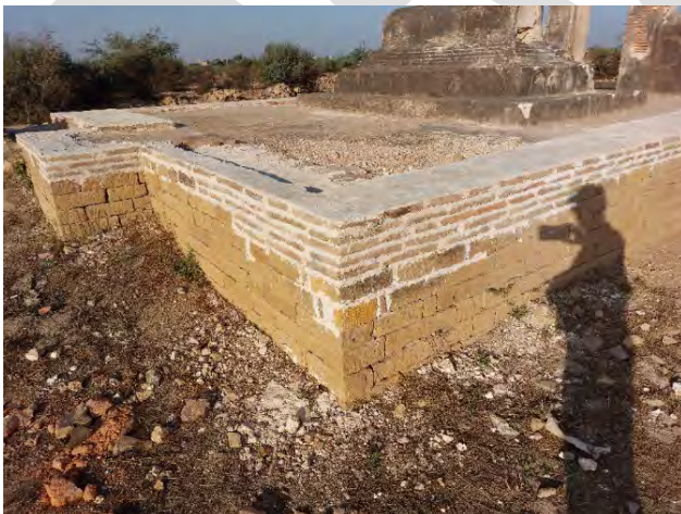
Figure 10 The work is generally well executed, with the correct materials, lime mortar created on site and the original bricks, or replacement bricks of the same dimensions and composition. However, the mortar could be colored to better blend in with the age-value patina of the lower masonry courses. This is a small detail, as time will add to the patina.
