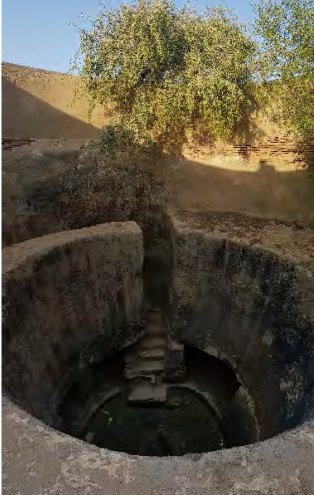
Figure 11 The impressive step well at the south of the site has been cleaned and can be used as a natural drainage. However, the historic channels leading into the well must be carefully investigated (Eppich)
