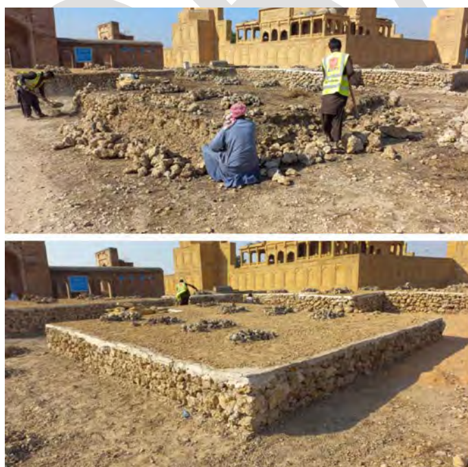
Figure 3 Restoration of a rubble masonry platform tomb near the monumental tomb of Isa Khan II that was damaged in the monsoon. Above, before, below after (Serfraz Nawaz)
