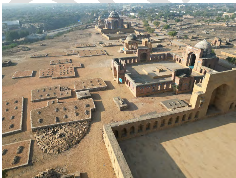
Figure 2 Overview of the Mungul period cluster near the main entry after improvements in drainage, cleaning of burned areas, and consolidation of the platform tombs (Eppich)
