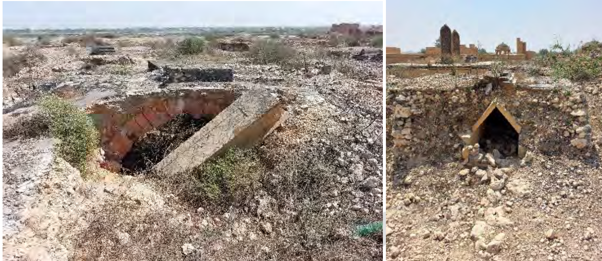
Figure 26 Other damages include the erosion of the platforms that expose the vaults of the tombs below.
