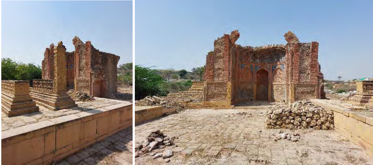
Figure 33 Left, the site has been cleaned and the bamboo scaffolding removed since the 2022 report, but Kashi tile and historic masonry consolidation must be immediately begun.
