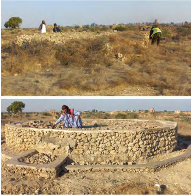
Figure 4 Restoration of an octagonal rubble masonry platform tomb just off the main road that was damaged in the monsoon. Above, before, below after (Serfraz Nawaz)
