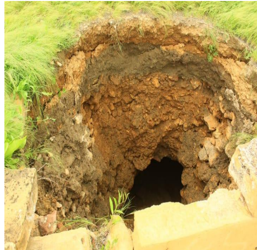
Rainwater penetrated inside the foundation and weakened the brick subsurface structure
