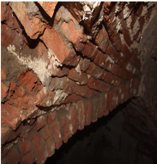
Rainwater penetrated inside the foundation and weakened the brick subsurface structure
