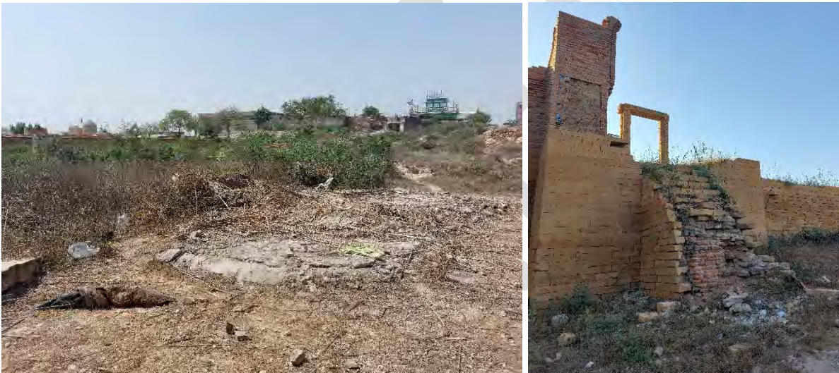
Figure 34 The bamboo huts have been dismantled and removed, but the site still requires significant cleanup. Right, the masonry entry steps and wall tops require consolidation.
