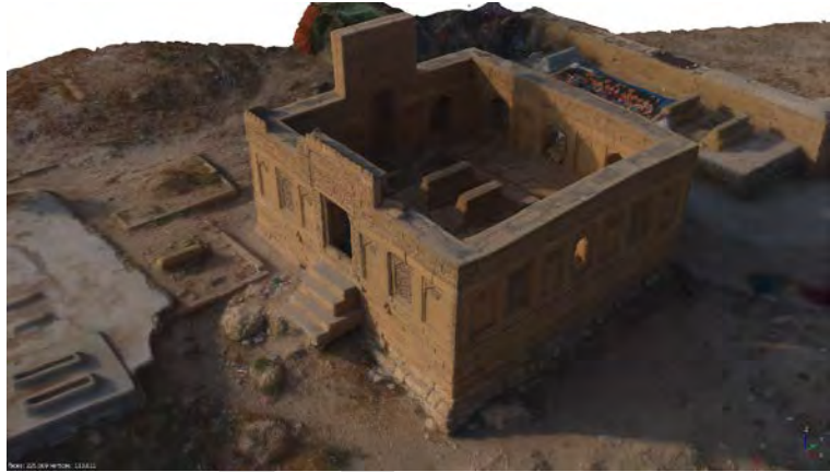
Figure 28 Continued erosion of the access steps and eastern boundary wall of the enclosure tomb of Badi Uz Zamman Tarkhan, left. Right, a 3D model was created of the enclosure tomb of Amir Habshad Bai to document the erosion.
