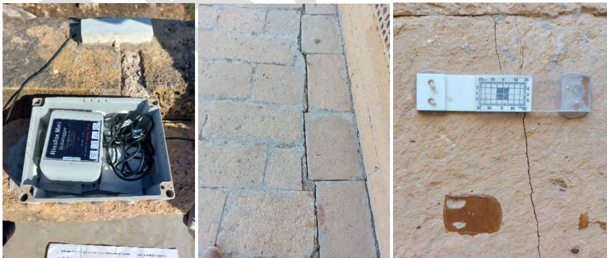
Figure 20 Left, the crack monitor, center the crack at the exterior base at the head of the slope, and a sketch of how water will enter this crack and erode the underlying soil. Figure 21 Right, polycarbonate crack monitors installed by Engineer Beckh were observed and showed a 1mm movement, but this was after the 2018 monsoon. Unfortunately, many crack monitors were lost (see below and right) and must be reinstalled for continued monitoring (Eppich).
