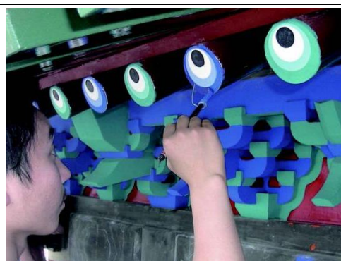
Fig. 3-11. Applying colored paintings to rafter ends
