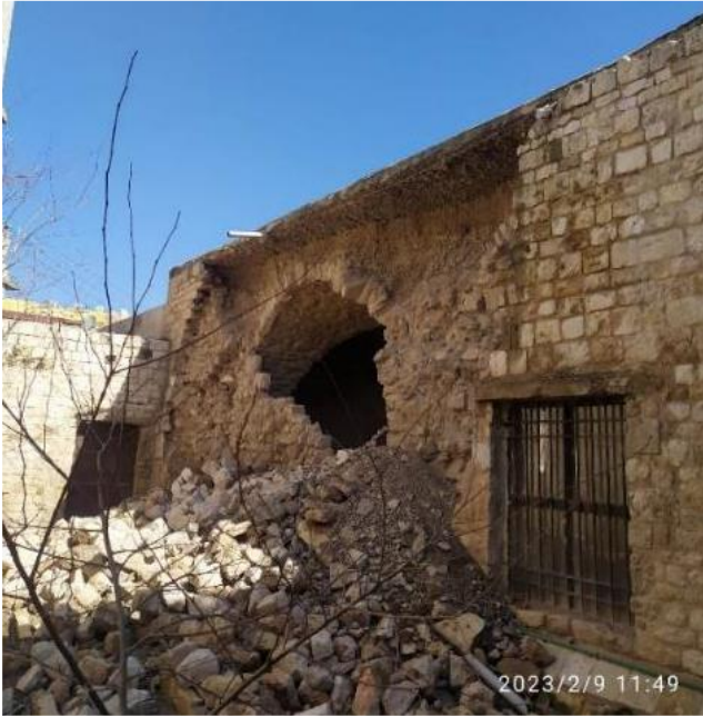
Al-Tawashi Mosque (Al-Qasila): Strengthening, consolidating and dismantling the facades and rebuilding in accordance with the original shape. Installing lime mortar and facade cleaning.
