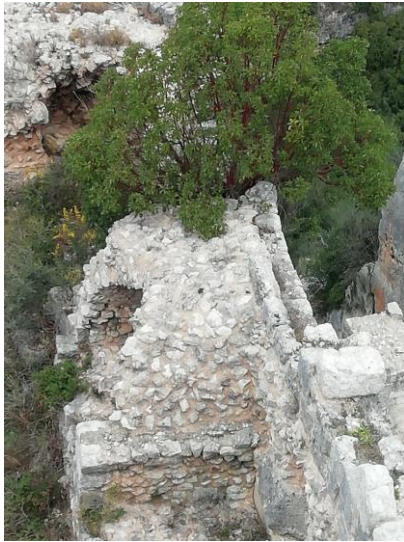
The damage at the defense's walls north of the Royal tower which is weak masonry walls without mortar had diagonal or inclined shear cracking.
