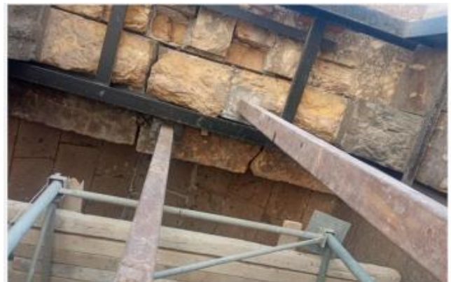
Installing temporary shore to control the lintel's stability.
