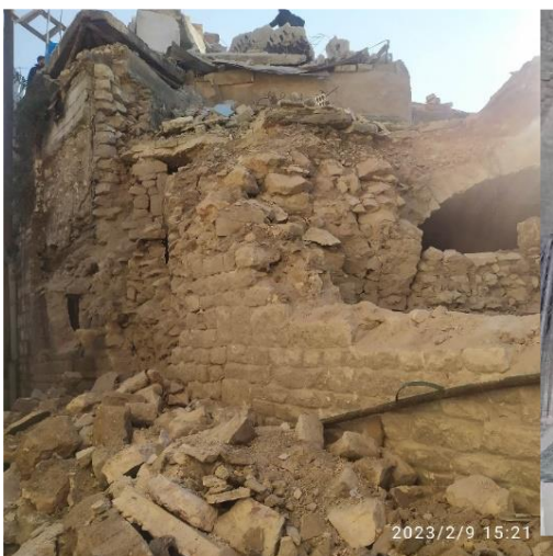
Al-Mayati Mosque (Al-Jaloum): Strengthening, consolidating and dismantling the facades and rebuilding in accordance with the original shape. Installing lime mortar and facade cleaning.
