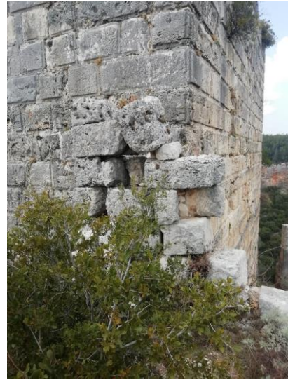
The damage at the defense's walls north of the Royal tower which is weak masonry walls without mortar had diagonal or inclined shear cracking.
