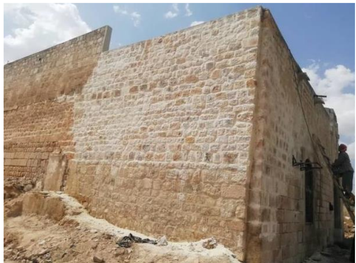
Al-Bawakeb Mosque (Al-Mashreqa): Strengthening, consolidating and dismantling the facades and rebuilding in accordance with the original shape. Installing lime mortar and facade cleaning.
