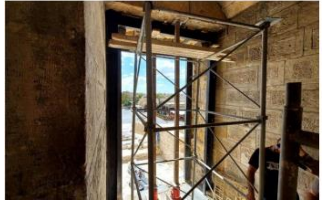
Installing temporary shore to control the lintel's stability.
