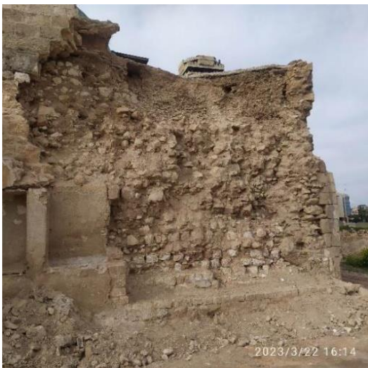
Al-Bawakeb Mosque (Al-Mashreqa): Strengthening, consolidating and dismantling the facades and rebuilding in accordance with the original shape. Installing lime mortar and facade cleaning.
