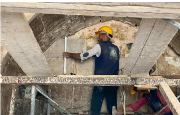
The temporary Consolidation of the vault carrying the stairs in the entrance doorway
