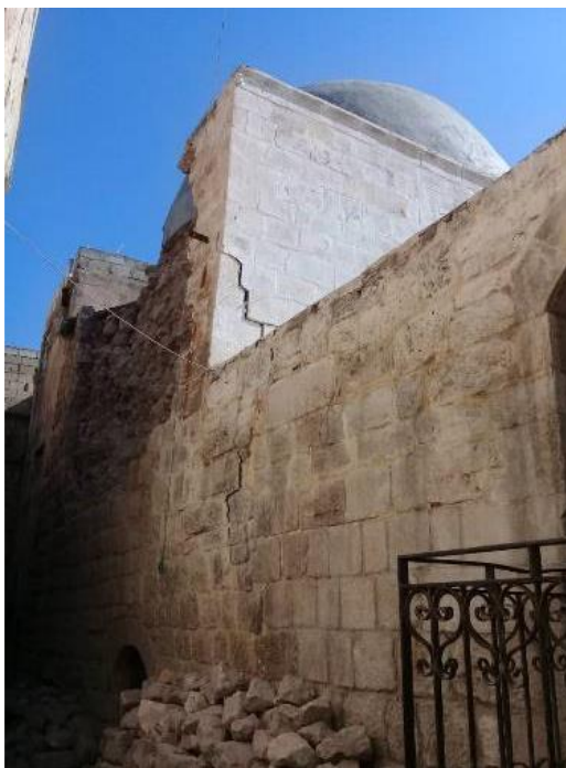
Al-Nour Mosque (Al-Jaloum): Strengthening, consolidating and dismantling the facades and rebuilding in accordance with the original shape of the facades. Installing lime mortar and facade cleaning.
