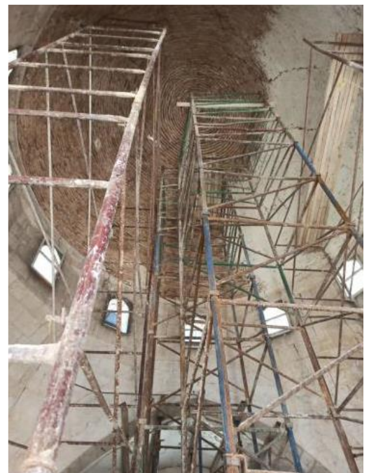
Minaret of the Tekkiyya Melawiyya - Al-Malkhana Mosque - (Bab Al-Faraj): Strengthening, consolidating and dismantling the dome of the minaret balcony with its supporting columns, and rebuilding damaged columns in conformity with the original form. Emergency strengthening work for the Hijazi Dome with initial injection of bonding materials in preparation for final restoration work.
