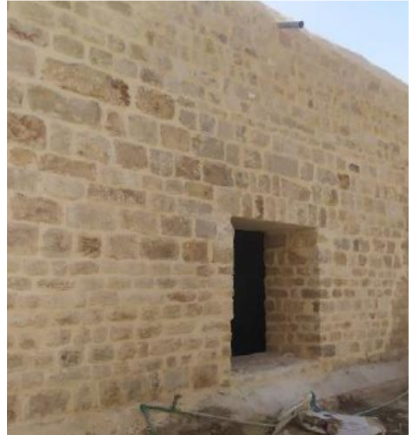
Al-Tawashi Mosque (Al-Qasila): Strengthening, consolidating and dismantling the facades and rebuilding in accordance with the original shape. Installing lime mortar and facade cleaning.
