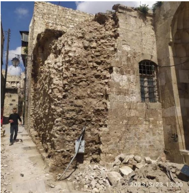
Kamaliyya Mosque (Al-Jaloum): Strengthening, consolidating and dismantling the facades and rebuilding in accordance with the original shape. Installing lime mortar and facade cleaning.
