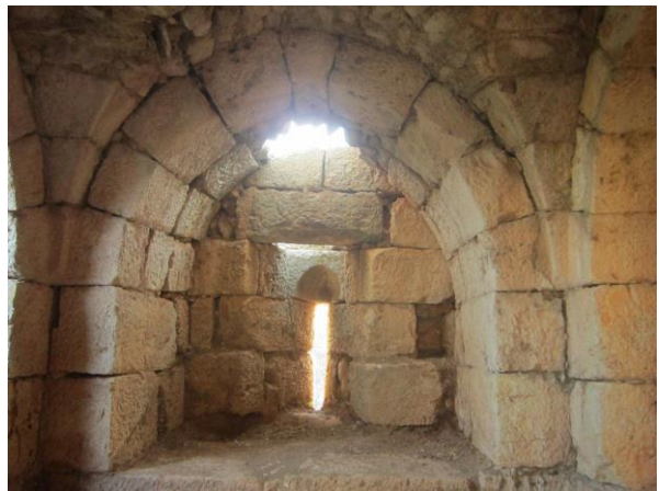
Cracks and chipped or loose stones, found all along the structure at the tops of openings.
