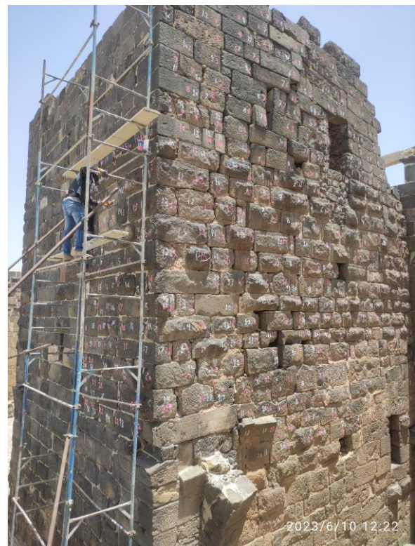
To help ensure the restoration and retention of structural integrity numbering and sorting the ancient stones and debris were developed.
