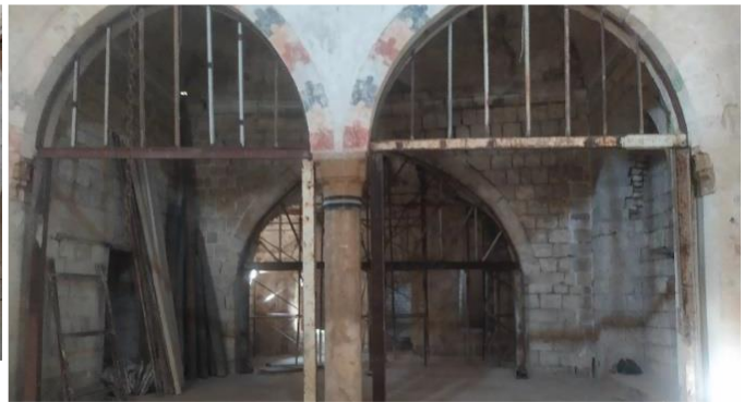
Al-Zawiya Al-Rifaiyya (Al-Bayada): Ambulatory strengthening works for the external facade with the arches inside the tribal area in preparation for the final restoration work
