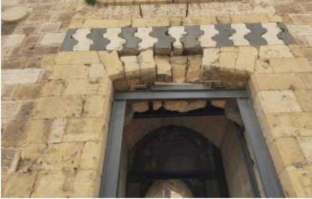
Dropped key stones of the entrance's lintel.
