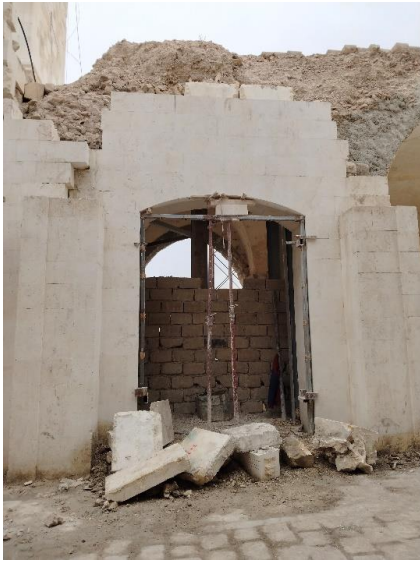
The damaged part of the western door was dismantled and rebuilt.
