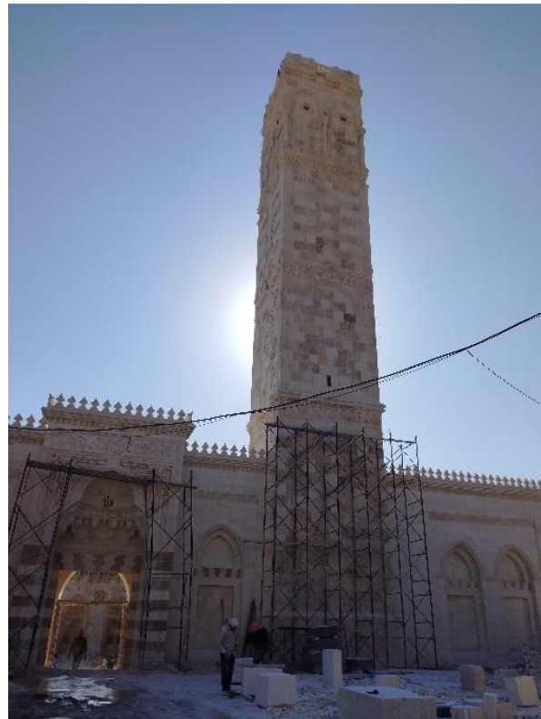
Restoration works were conducted on the outer western wall and the ceilings of the western and northern peristyle in addition to dismantling the earthquake-damaged part of the outer western wall in accordance with the agreed-upon study.
