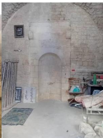
Al-Mayati Mosque (Al-Jaloum): Strengthening, consolidating and dismantling the facades and rebuilding in accordance with the original shape. Installing lime mortar and facade cleaning.
