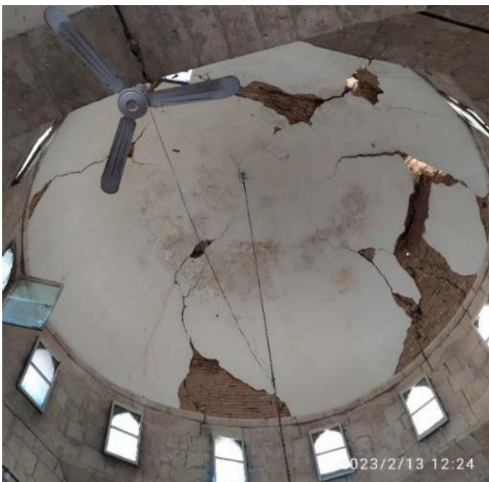
Minaret of the Tekkiyya Melawiyya - Al-Malkhana Mosque - (Bab Al-Faraj): Strengthening, consolidating and dismantling the dome of the minaret balcony with its supporting columns, and rebuilding damaged columns in conformity with the original form. Emergency strengthening work for the Hijazi Dome with initial injection of bonding materials in preparation for final restoration work.
