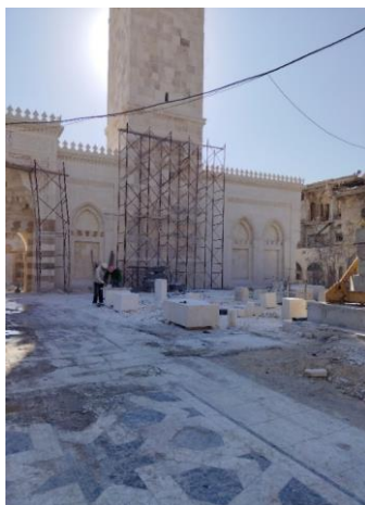
The rooms next to the minaret were rebuilt as it were before collapse with the ceilings and the crenel decoration on the main façade.
