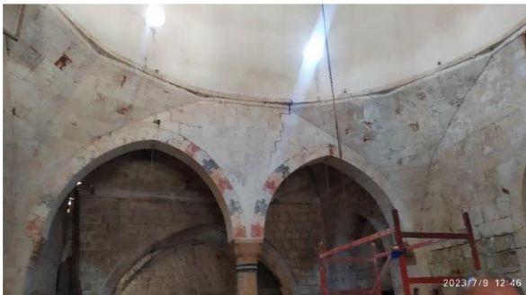
Al-Zawiya Al-Rifaiyya (Al-Bayada): Ambulatory strengthening works for the external facade with the arches inside the tribal area in preparation for the final restoration work
