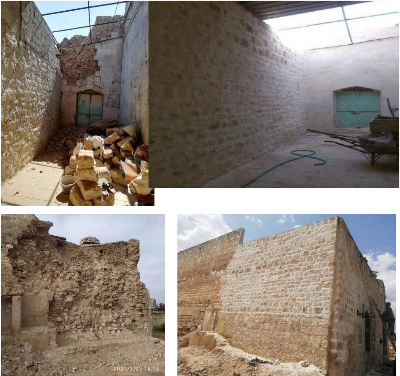
Al-Bawakeb Mosque (Al-Mashreqa): Strengthening, consolidating and dismantling the facades and rebuilding in accordance with the original shape. Installing lime mortar and facade cleaning.
