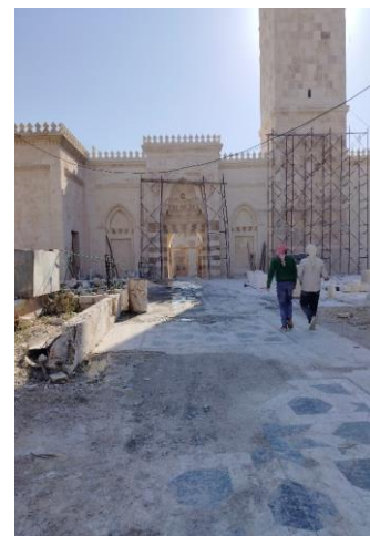
The façade of the main entrance was rebuilt along with the stalactite façade and the crenels.
