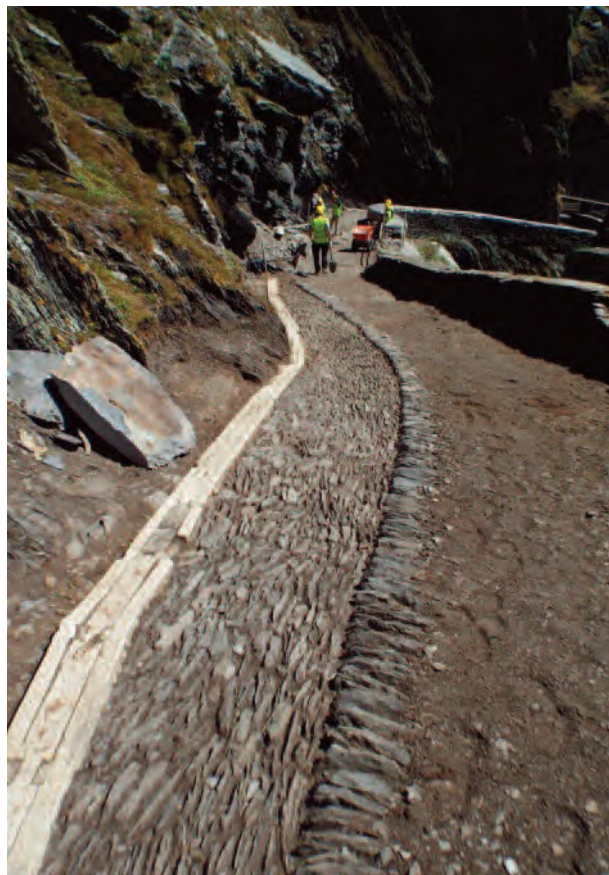
Pl. 31 The Upper Lighthouse Road, after excavation, showing the original road surface, drains and an electrical conduit inserted in the early twentieth century.
