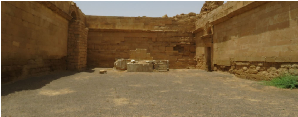
Figure 8: Temple of Allat, coarse sand laid over geotextile © UNESCO / M. Shaer
