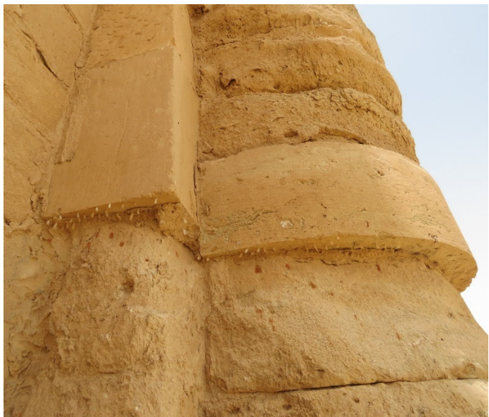
Fig 117: Erosion of original stone masonry adjacent to next to a previous modern intervention ©UNESCO/M.Shaer
