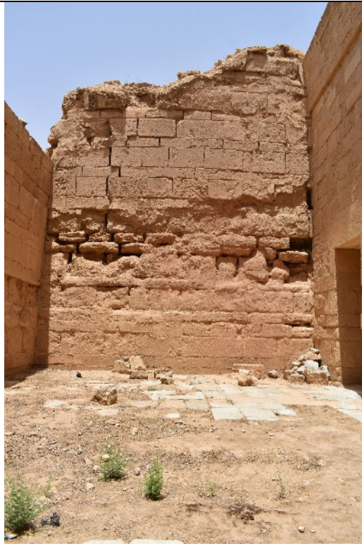
Figure 115: Deep masonry erosion ©ICOMOS/Y.Makaroun
