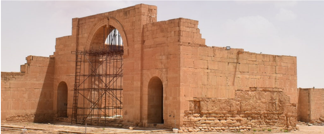
Figure 12: Temple of Samya, installation of propping © ICOMOS / Y. Makaroun
