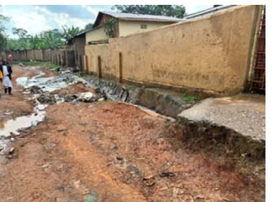
Sanitation issues in the buffer zone
