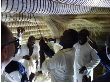
Traditional builders finalizing the ceiling
