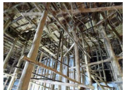
Scaffolding in the interior
