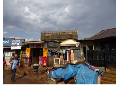
Multi-storey building under construction inside the buffer zone
