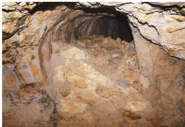
● Photo c1-2 Connection vent (blocked with waste rocks and clay except for the upper part)
