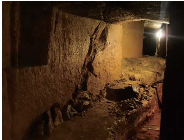
● Photo c2-3 Breakthrough point by mining from the both sides
