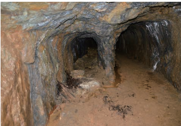
● Photo c1-1 Ventilation tunnel (right) and main tunnel (left)
