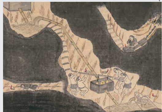
● Figure 34 Dutch-style water pump, "Kinzan shikioka kasegikata zu" (Picture of mining method in mines (inside and outside)) [Property of Kyushu University Museum]
