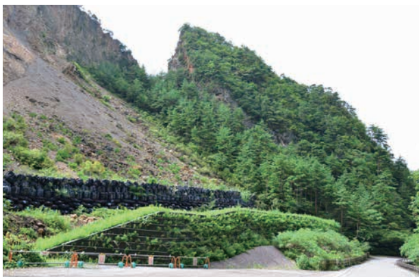
● Photo 3-2 Countermeasure against rockfall with pro-environmental construction method (Geo Rock Wall method)
