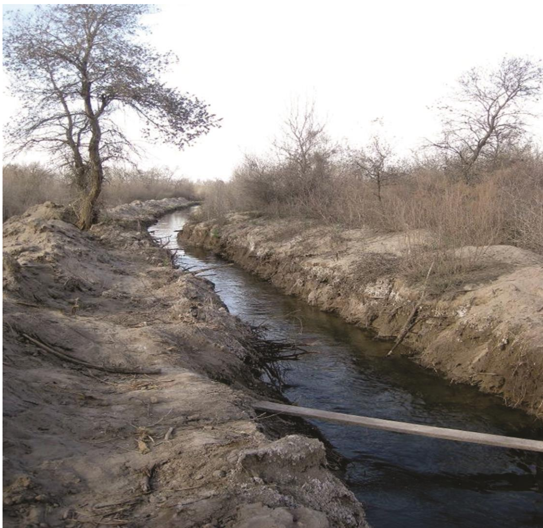
A branch from the main channel, designed to feed the floodplain lakes of the Tigrovaya Balka Nature Reserve
