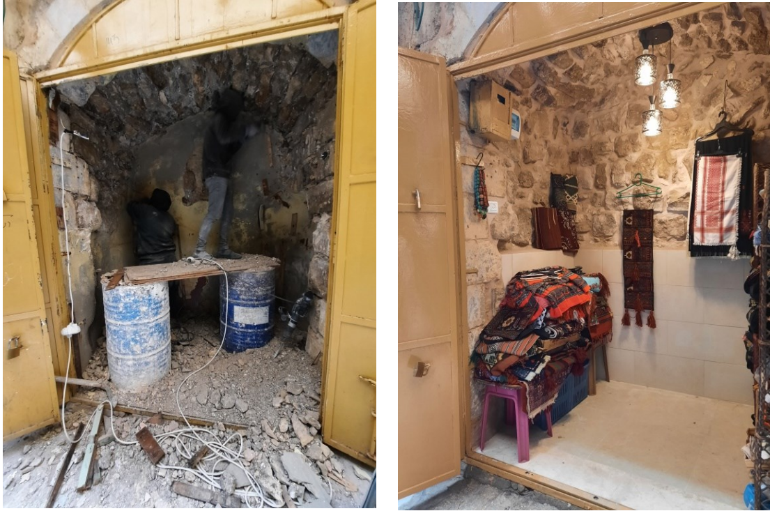
Figure 5: Rehabilitation of commercial stores (before &after)
