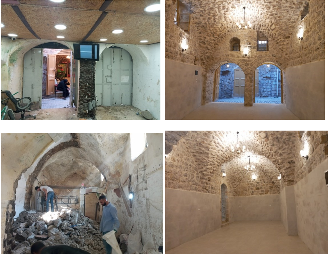
Figure 4: Rehabilitation of commercial stores (before & after)
