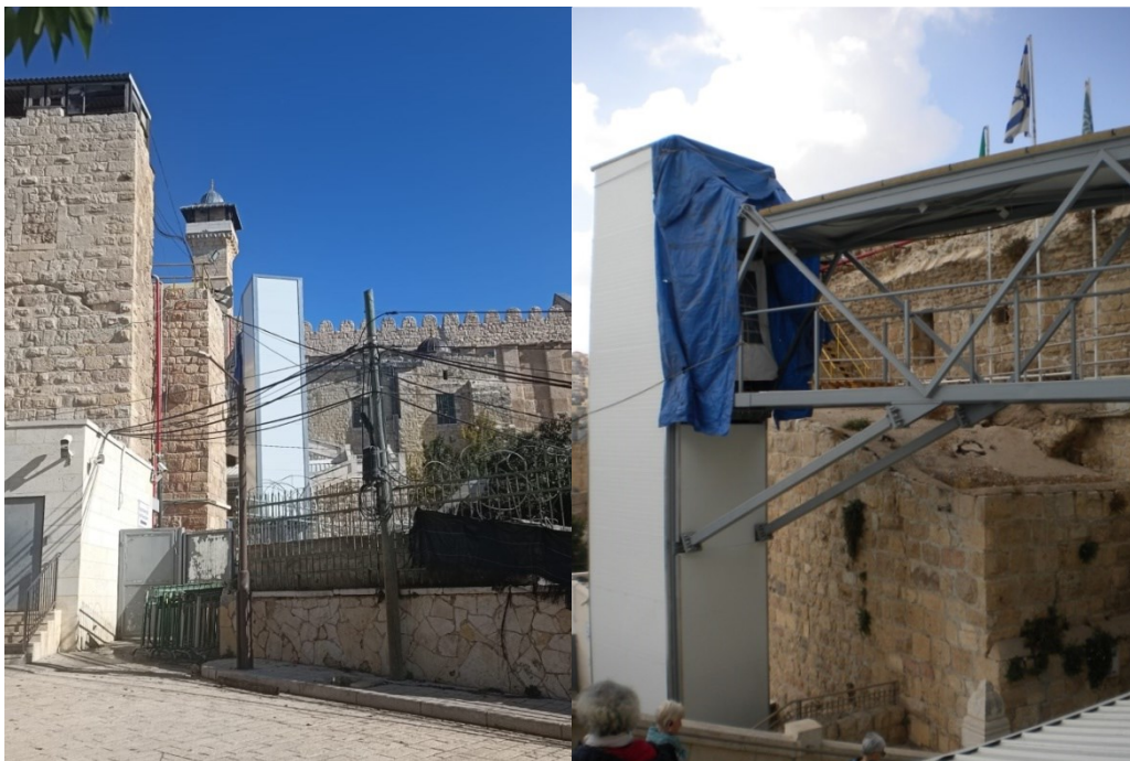
Figure 13: The construction of the electric elevator
