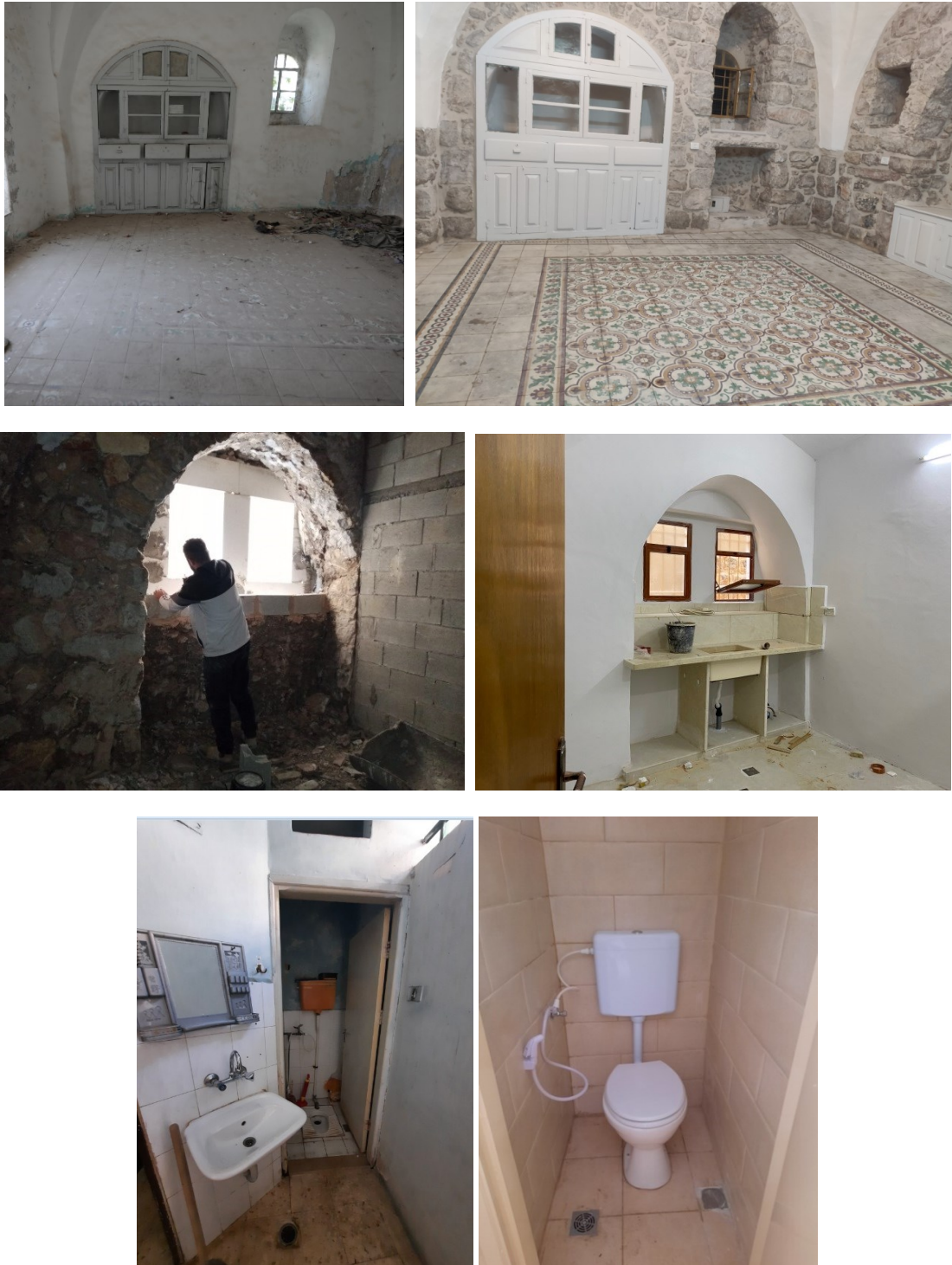
Figure 2: Regular Maintenance of historic buildings (before and after)
