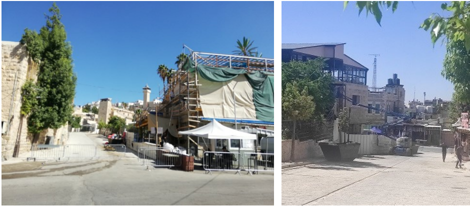
Figure 19: Constructions of new concrete-stone stories in front of the Ibrahimi Mosque
