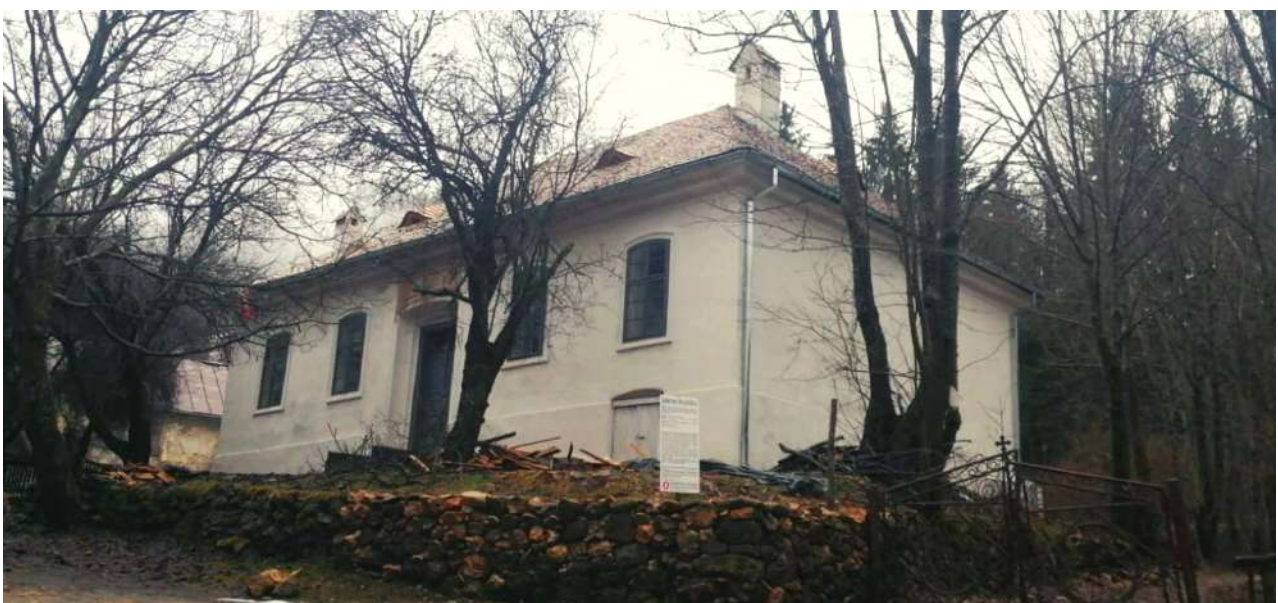
_photos: before and during repairs / rosiamontana.community (partner).
