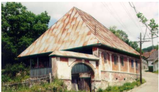
▶ The former maternity ward
