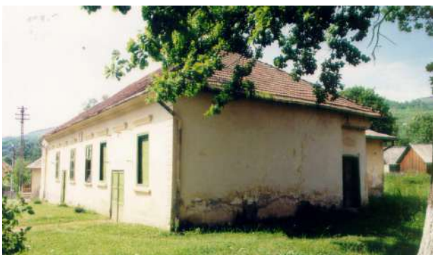
▶ The former cinema
