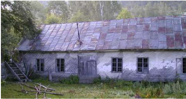
▶ The former slaughterhouse
