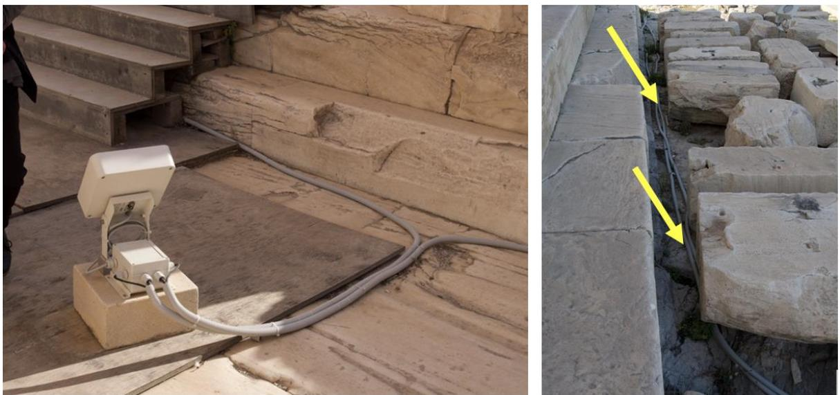
Figure 11 Light projectors for the lighting of the Acropolis, located around the Parthenon.
