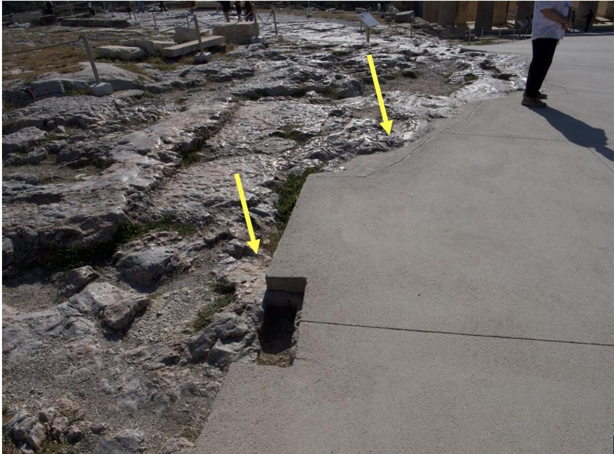
*Figure 3 Different treatments of the pathway profiles*
