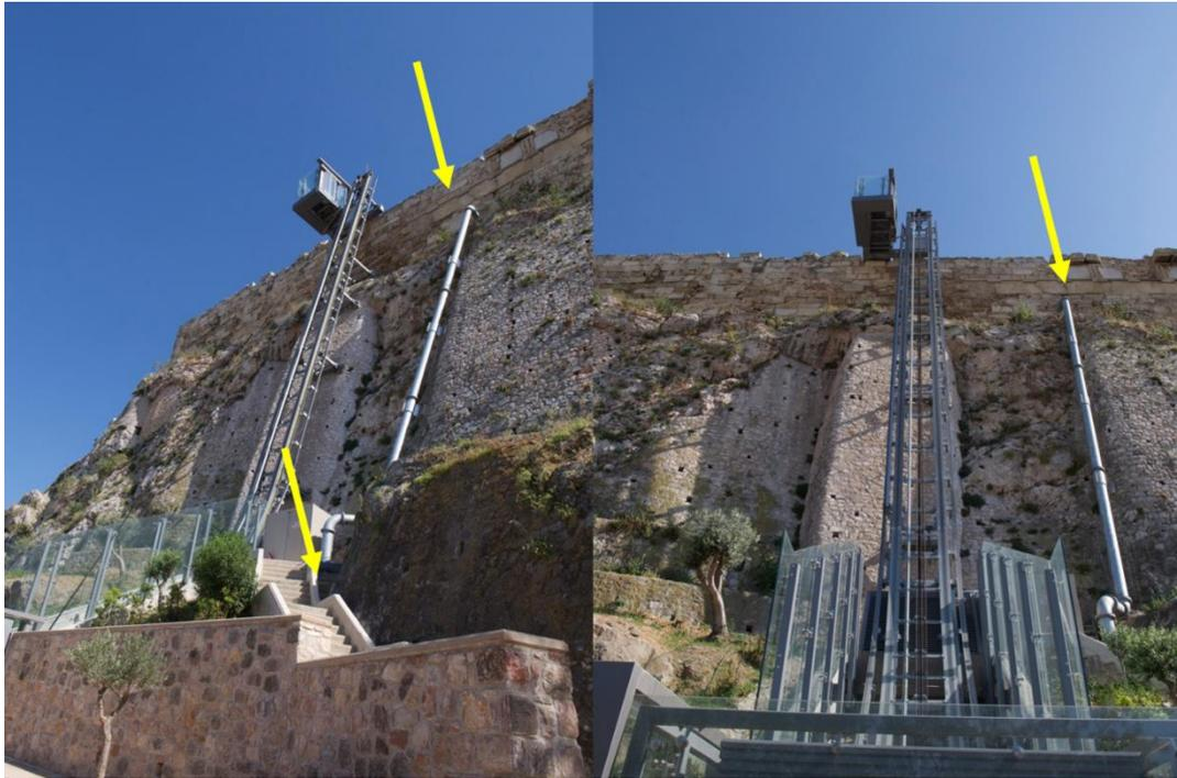
*Figure 4 North-West side drainage plumbed to the exterior downspout next to the elevator*
