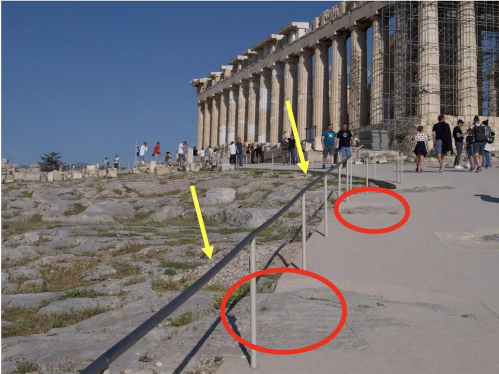
Figure 12 Handrail specifically designed for the Acropolis site to guide blind people. The handrail integrates information for visitors in Braille. At the moment, the handrail crosses several archaeological windows that could become a danger for certain categories of visitors, and especially for blind people.
