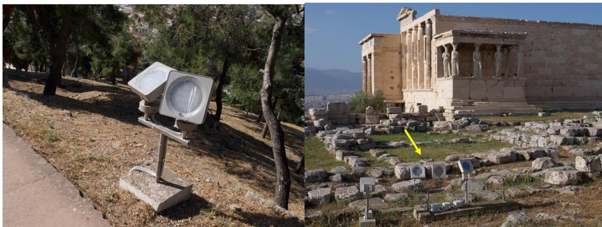
*Figure 9 Light projectors for the lighting of the Acropolis, located within the site.*
