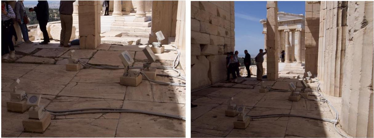
Figure 10 Light projectors for the lighting of the Acropolis, located within the Propyleae.
