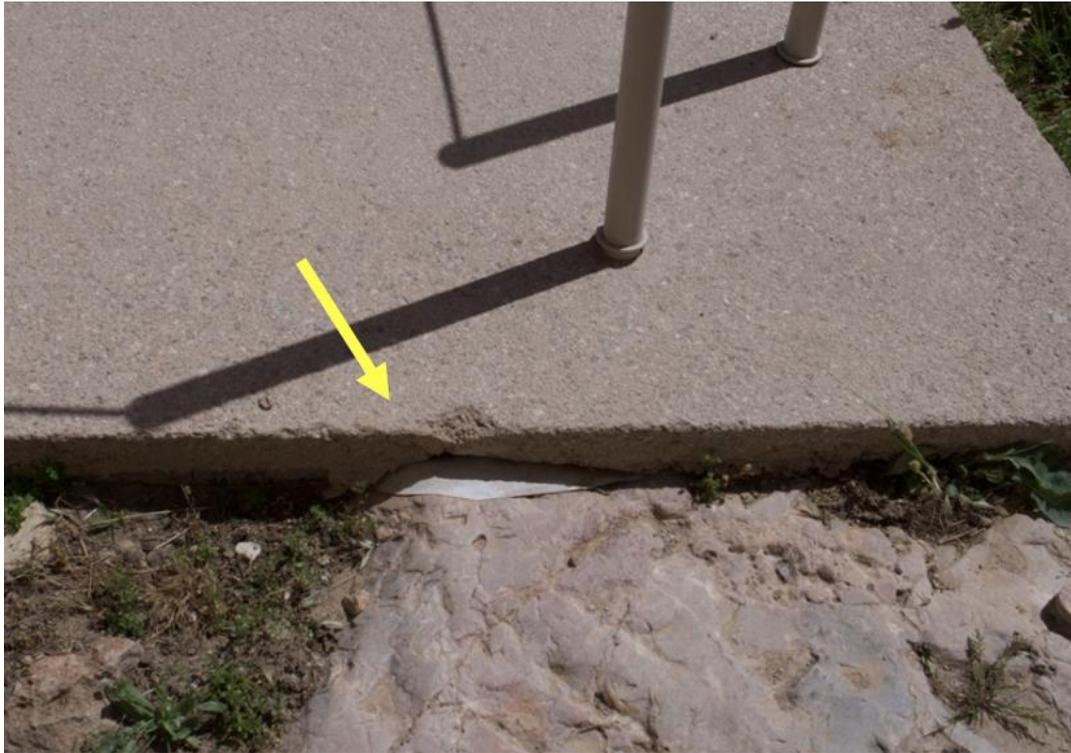
*Figure 5 PVC layer isolating the surface of the rocks from the paving of the path and ensuring reversibility.*
