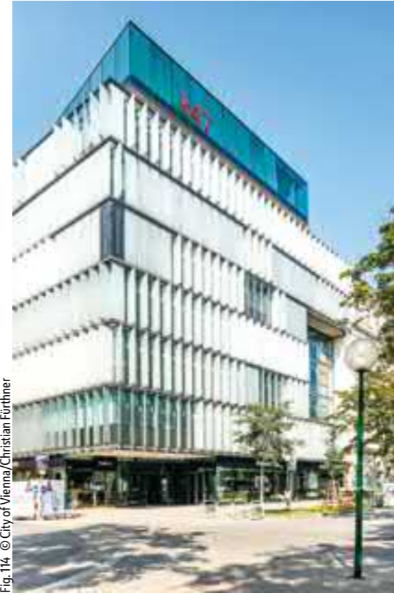
Office and commercial building K47 at Franz-Josefs-Kai (2003, Henke Schreieck Architekten) (Fig. 114)
