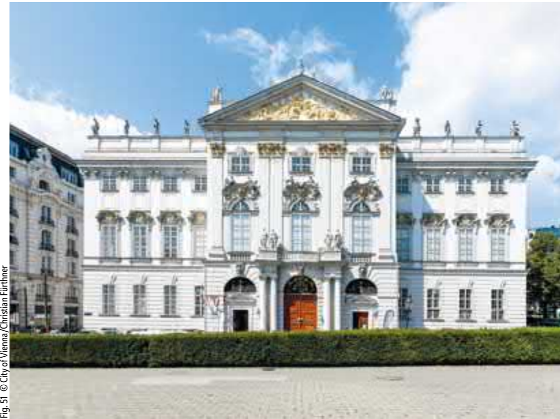
The Palais Trautson was built from 1710 onwards according to plans by Johann Bernhard Fischer von Erlach. Originally situated on the edge of the suburb, the garden palace now houses the Ministry of Justice. (Fig. 51)
