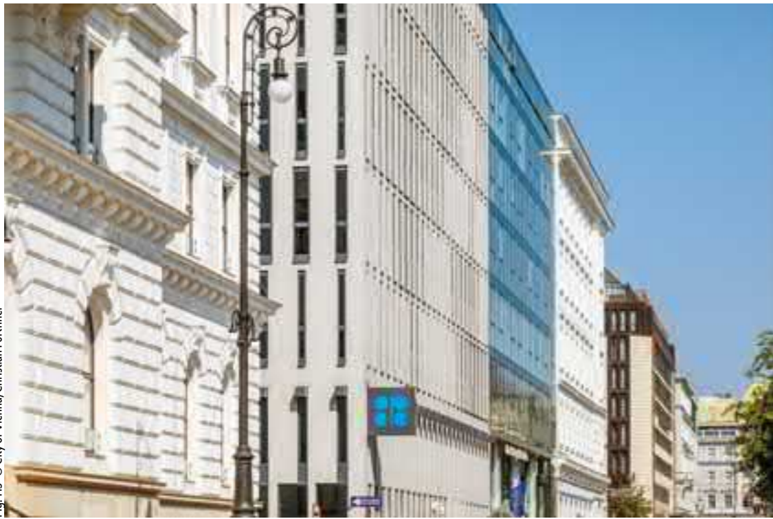
OPEC headquarters i n Wipplingerstrasse (2009, HD Architekten (Fig. 113)
