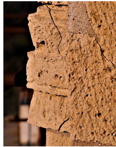
Fig. 47. West arm – W-S corner: Fractures of structural and decorative elements
