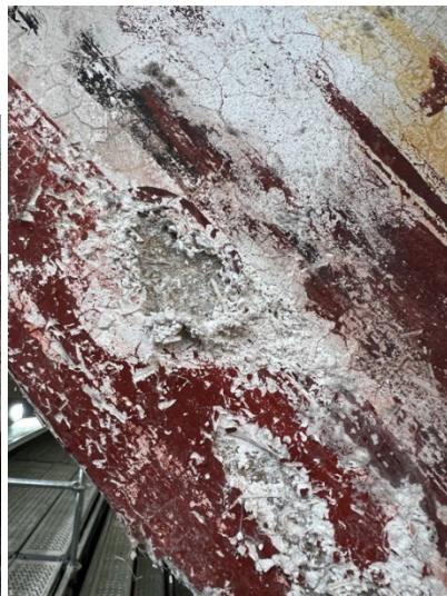
Fig. 32,33. Areas with severe plaster decay under the northwest pendentive
