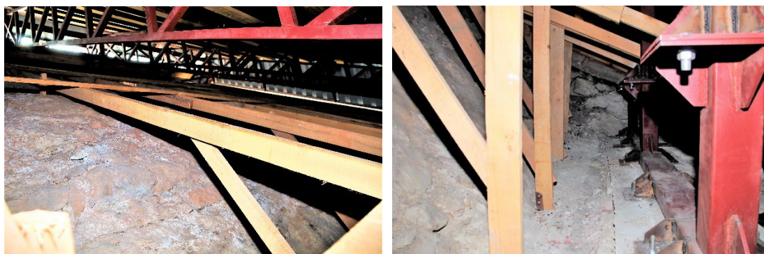
Fig. 23. The iron truss system supporting the new temporary roof covering the extrados of the west arm
