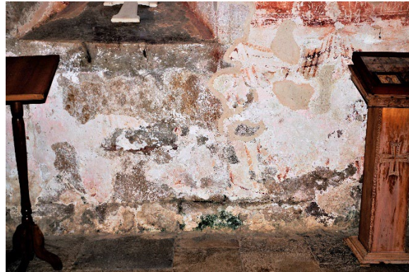
Fig. 61. St. George: exterior view, north side. Detail of the visible rising damp (by ReStruere)
