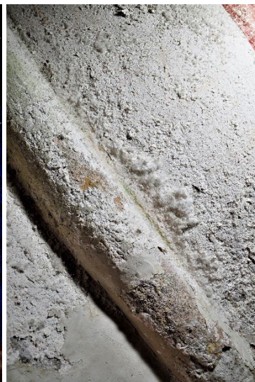
Fig. 50. North arm – frontal arch: intensive presence of nitrates on the arch surface
