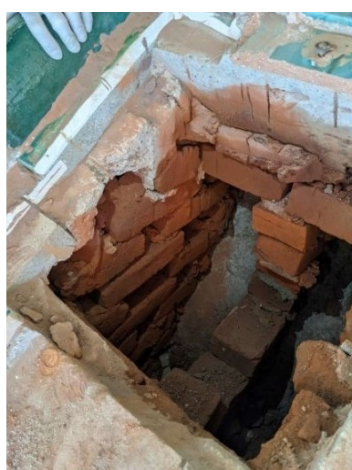
Fig. 10. Survey N3 on the east slope of the apsis roof (pitch N13), view from the north-east: plenty of moisture under the glazed tiles (Georgian team report, 1/2022)
