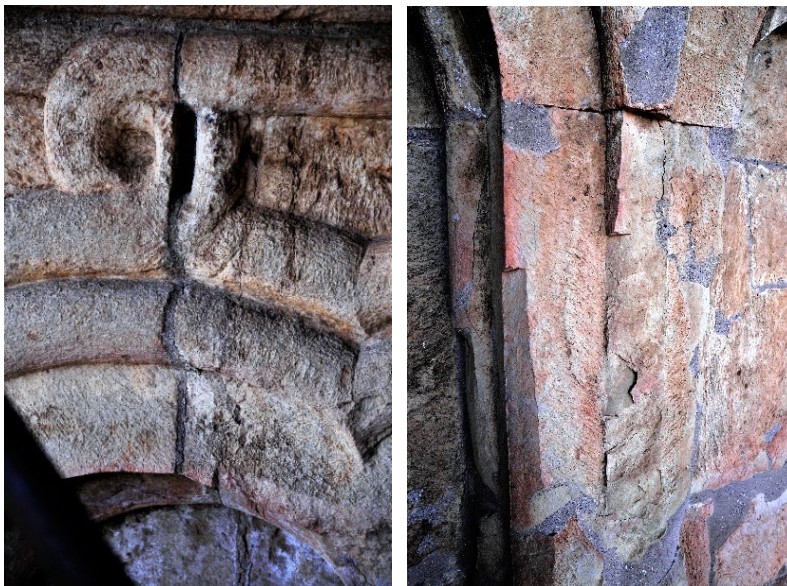
Fig. 53, 54. North arm – west façade: open joint cracks, fabric detachment and salt crystallization
