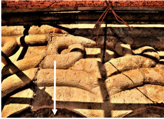
Fig. 44. West arm – south façade: Shifting of structural – decorated ashlars
