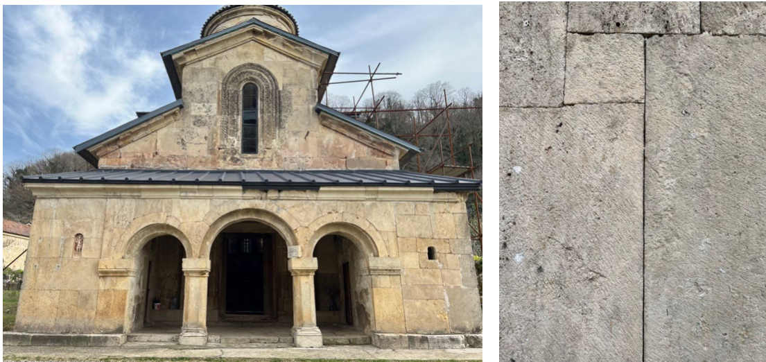
Fig. 58, 59. View of the façade of the Church of Saint George: need for infills in external stone joints, to avoid water penetration
