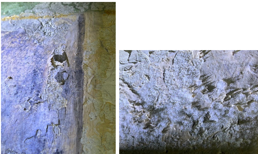
Fig. 29, 30. Detachment of paint layer and salt efflorescences in the northern wall of the west wing
