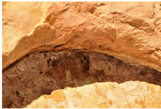
Fig. 44. West arm – south façade: Shifting of structural – decorated ashlars
