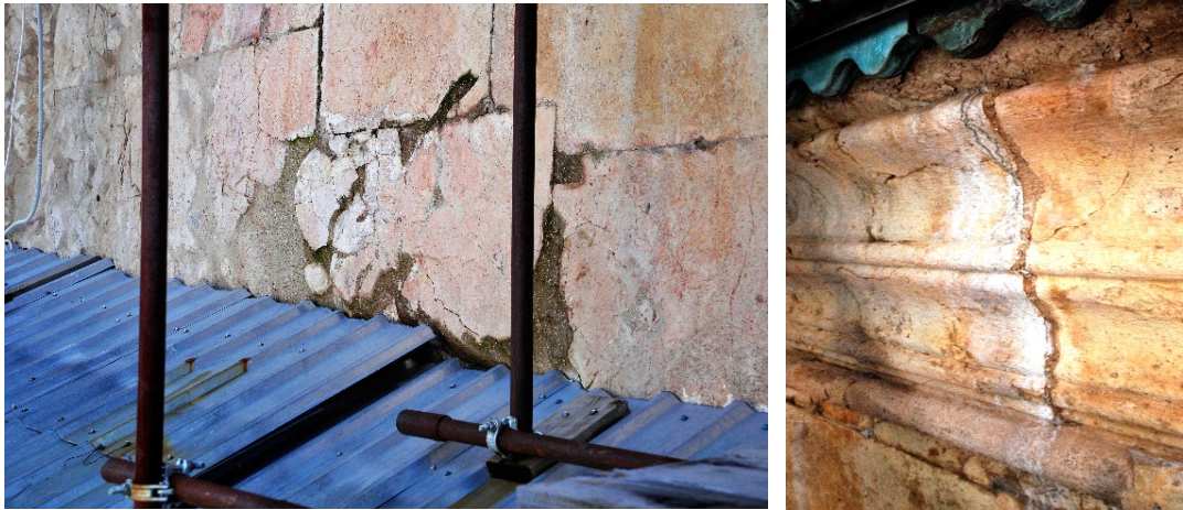
Fig. 51, 52. Condition of the north façade near to north arm – recent humidity on the joints' mortar and salt crystallization
