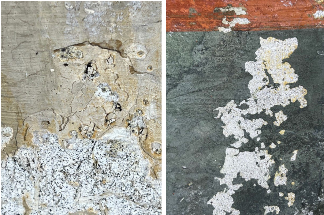
Fig. 27, 28. Subflorences and paint layer detachment in the southern wall of the west wing
