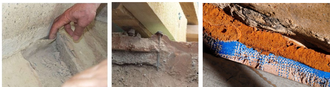
Fig. 12. Incorrect installation technique: a short strip of insulating material / nails penetrating the liquid insulated mortar (by ReStruere)
