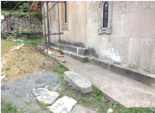
Fig. 61. St. George: exterior view, north side. Detail of the visible rising damp (by ReStruere)
