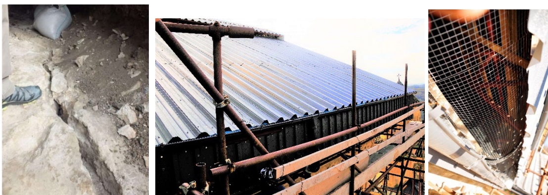
Fig. 20. Southern wall of west arm. Longitudinal crack on the top of the wall (by ReStruere)
