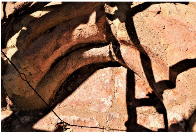
Fig. 46. West arm – south façade: Salt presence on the joints
