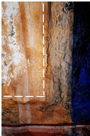
Fig. 48, 49. North arm – west wall: shifting of the building ashlars
