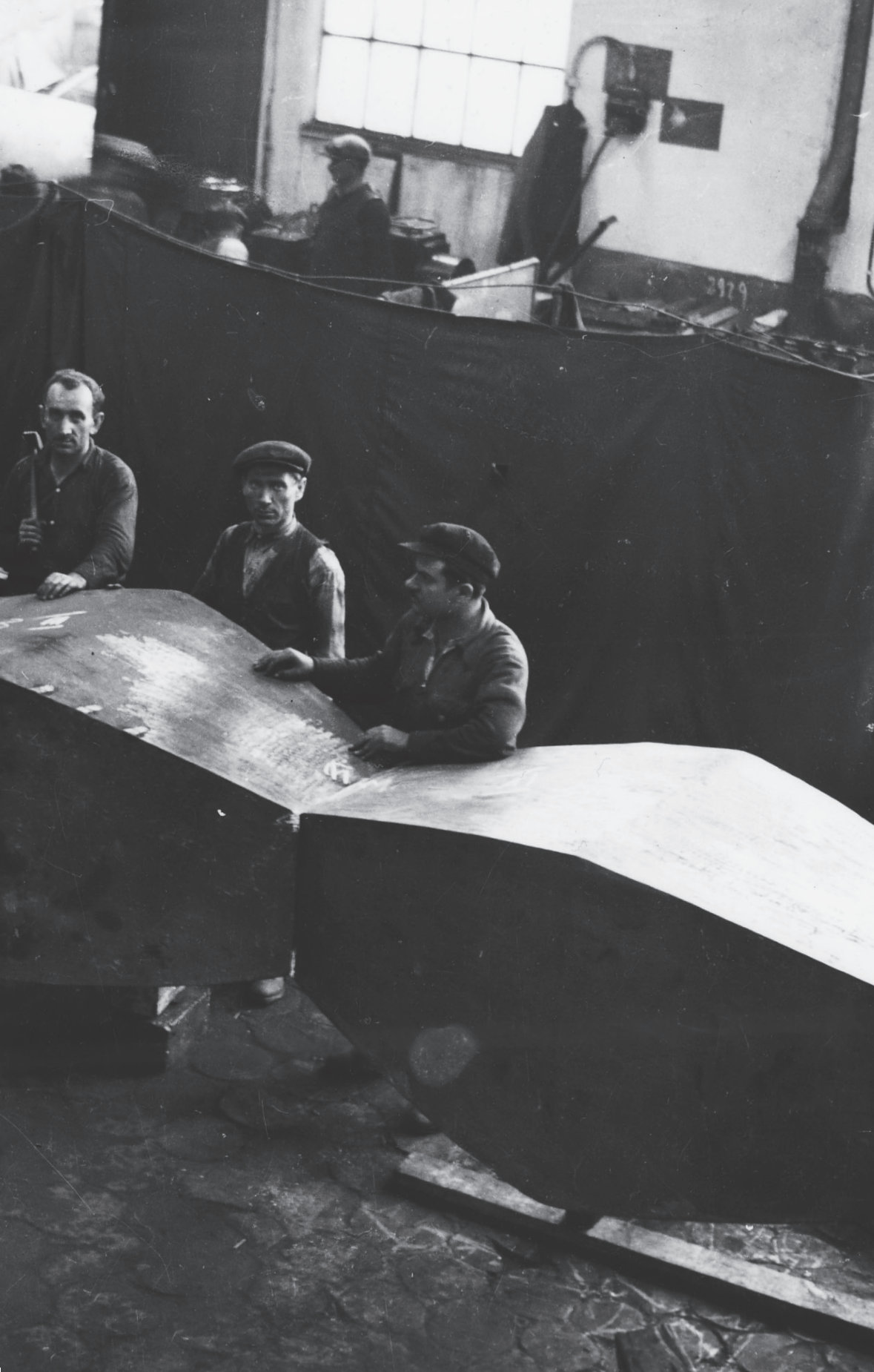
Test fitting of the Endless Column in the Petroșani Central Workshops. 1937 (INP Archive)
