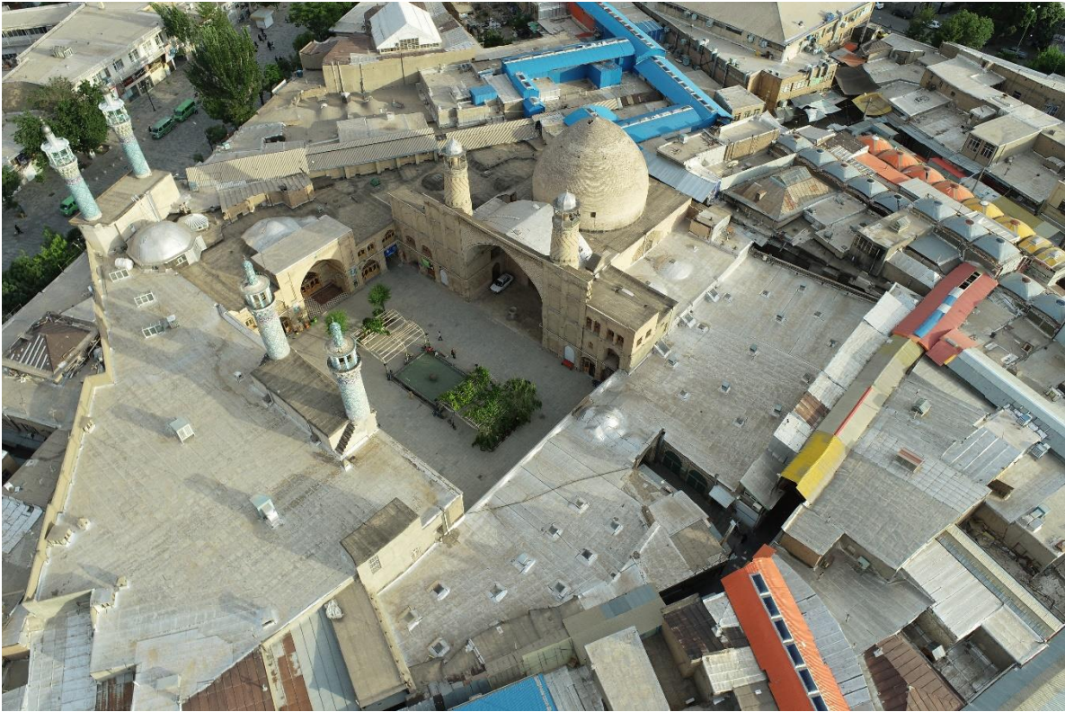
Figure. 4: View of the Masjed Jame. (Source: Ali Eqra)
