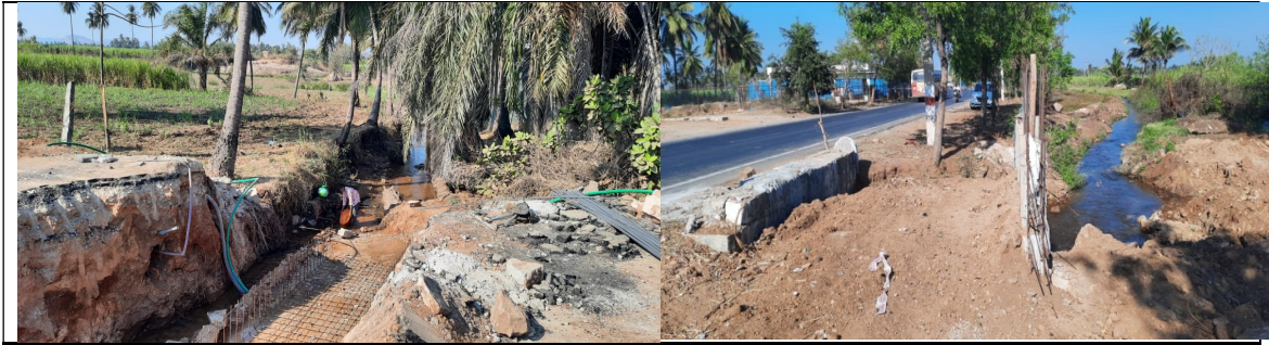
Road Widening Near Kamalapura Tank
